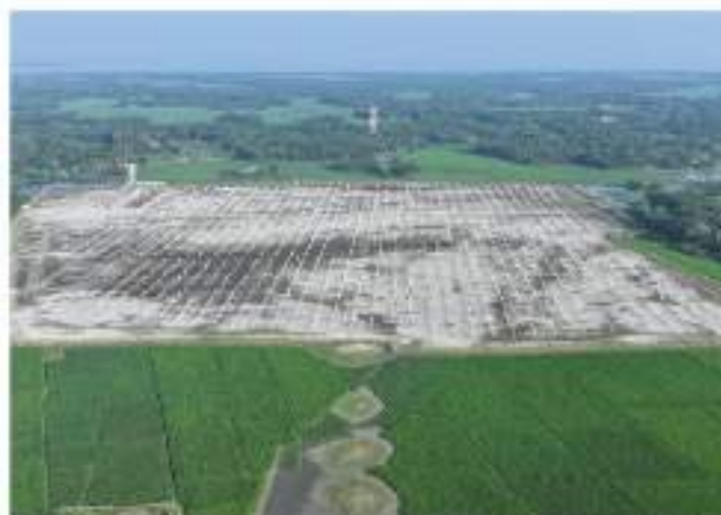
Ongoing Solar Power Plant in Monpura Islands, Monpura, Bhola.
