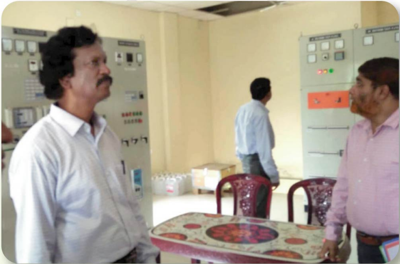
Managing Director, WZPDCL Visiting Newly Constructed S/S at Bhola
