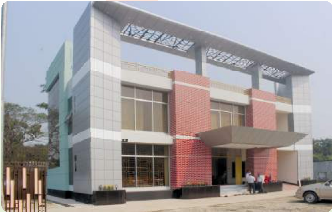
Newly Constructed RE office Building, Fultola, Khulna.
