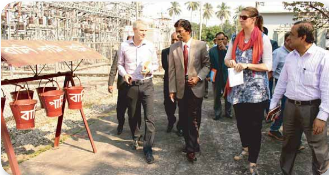
Managing Director, WZPDCL and representative of KfW (Germany) visiting 33/11 KV khayertala substation Jessore for upcoming SCADA Project
