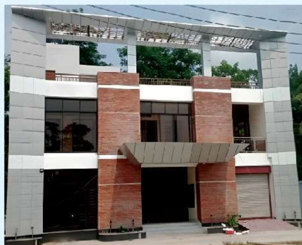
Kathalia electric supply office building
