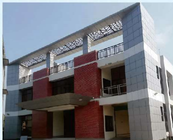
Charfassion electric supply office building
