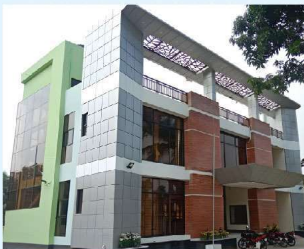
Kotchandpur electric supply office building
