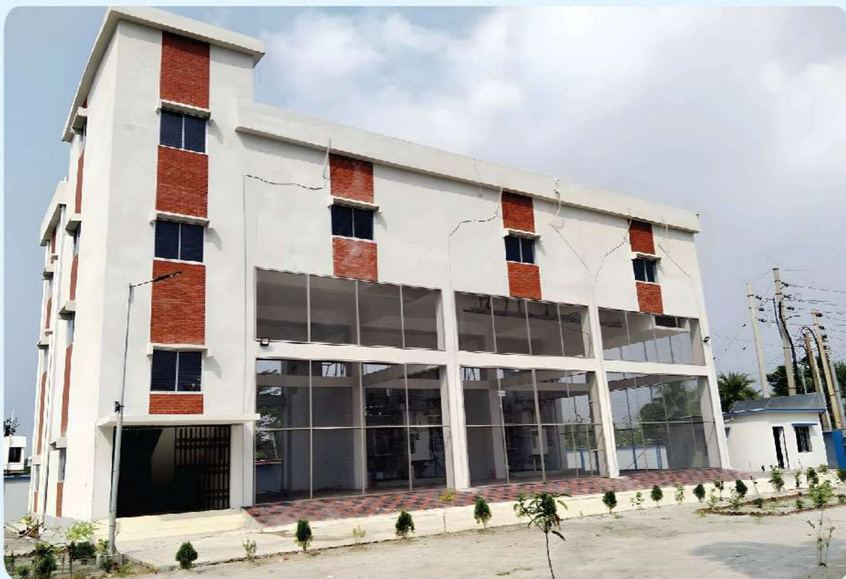
Newly constructed Sonadanga , S&D-4, Khulna 33/11 KV, 2×20/26.66 MVA GIS Substation by EUPDSP.
