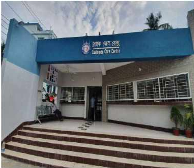
Newly Constructed Vending Station cum Customer Care Centre
