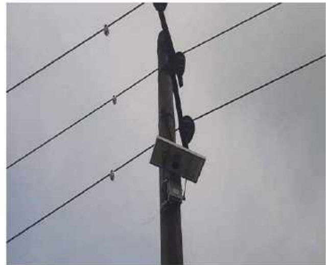
FPIs Installed in Patuakhali-Payra 33 kV Line
