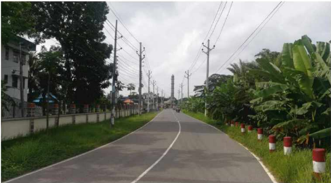
Newly constructed Shariatpur 33 kV source Line by EAUPDSP
