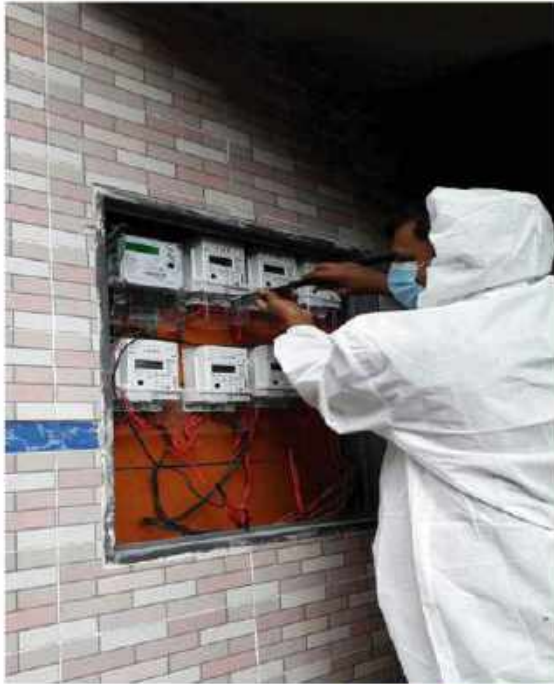
Installation of Smart Pre-payment Meter
