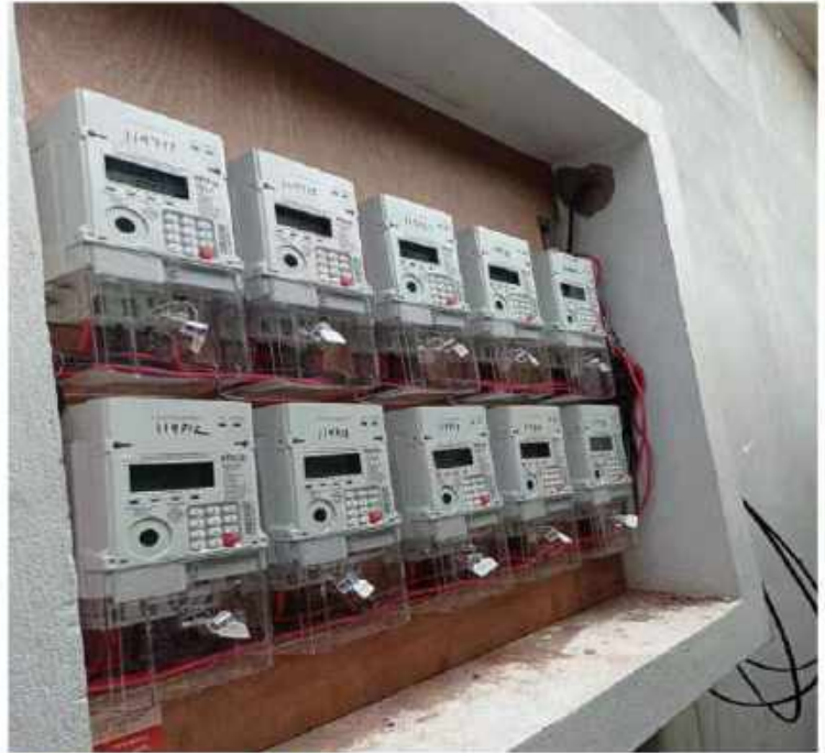
Installation of Smart Pre-payment Meter
