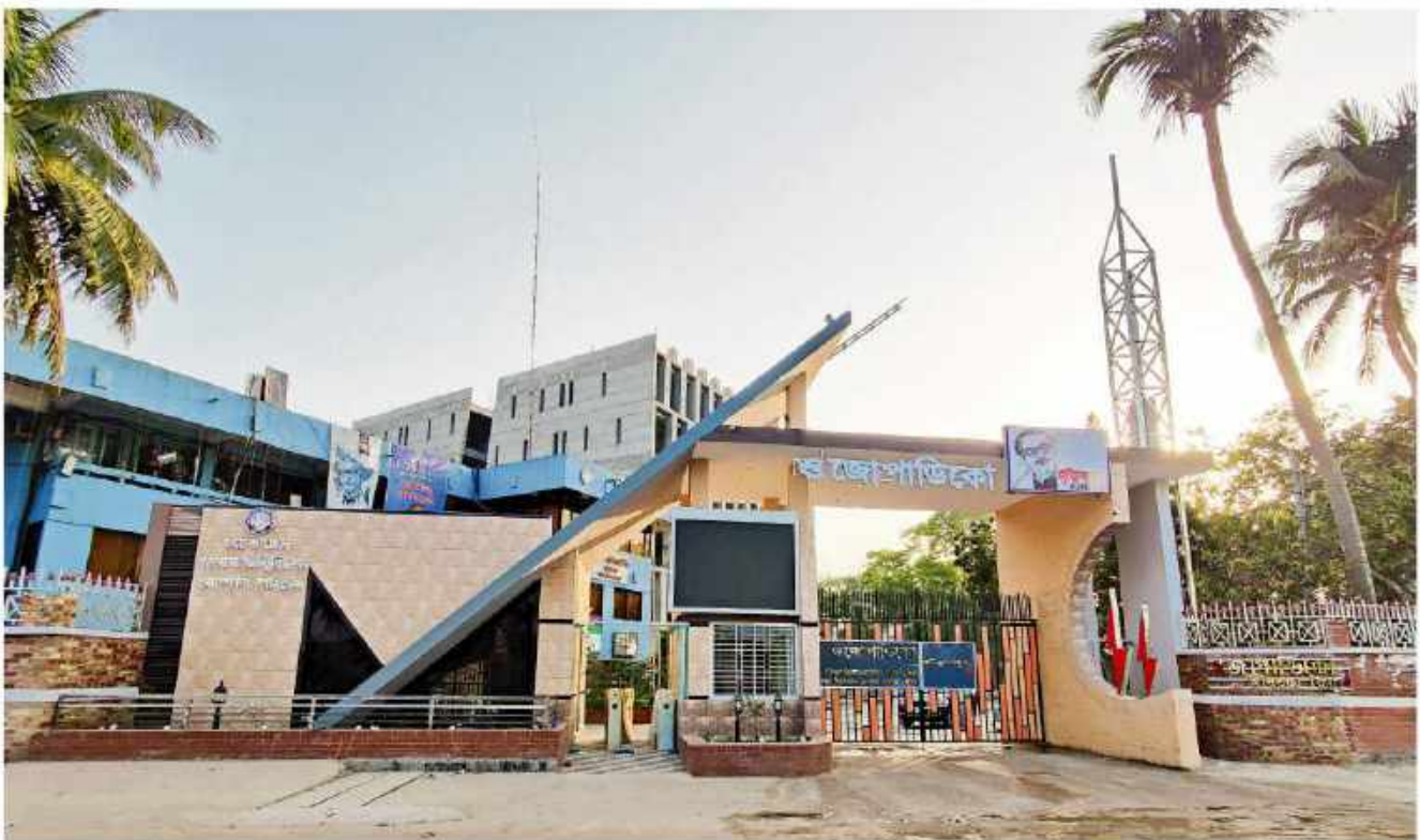
Newly constructed Head Quarters Main Gate by EAPDSP
