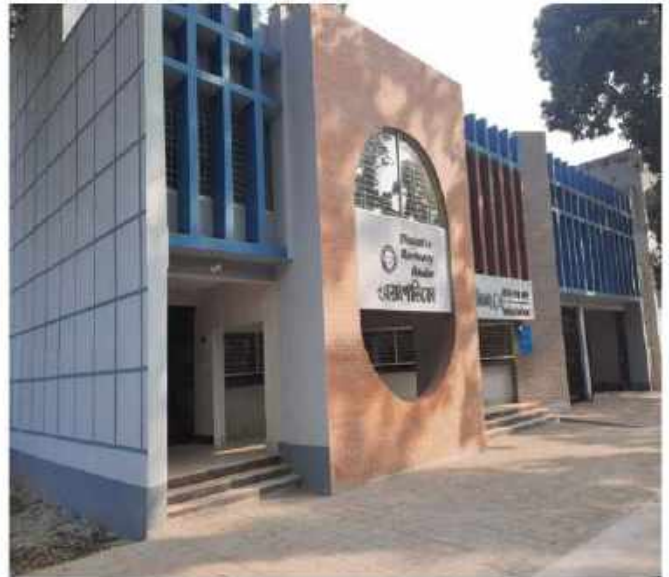
Newly Constructed Disaster Recovery Centre at Jashore
