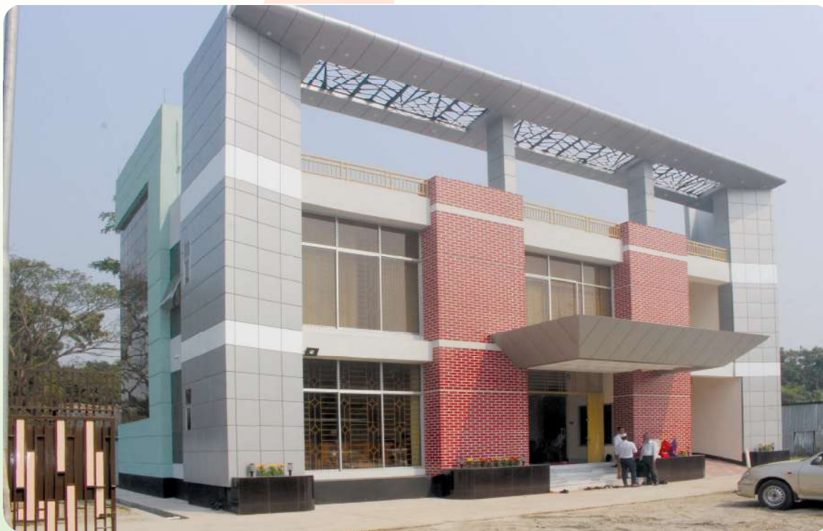
Newly Constructed RE office Building, Fultola, Khulna.
