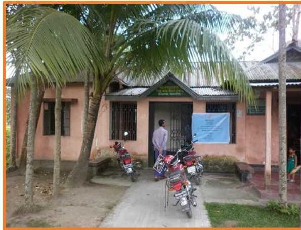
Photograph 5.1: Site Office at Ishwarganj Upazila
