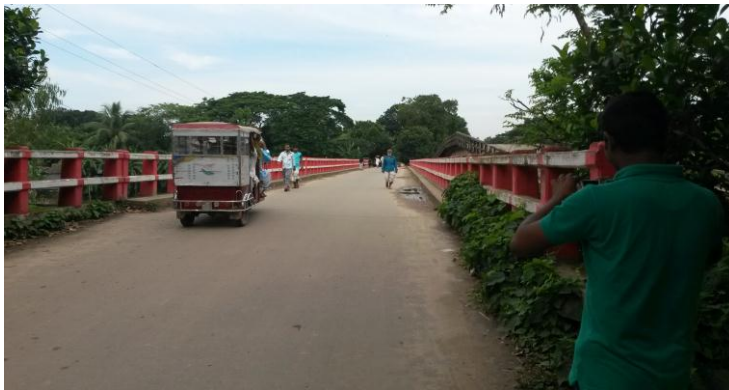
Plate-1: Bridge on Kalagachia Channel (Paharia River) at Shibpur Paurashabha at Narshingdi.
