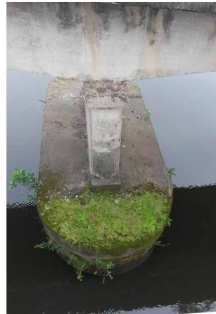
Plate-2: Pire of an abandoned Bridge on Kalagachia Channel (Paharia River) at Shibpur Paurashabha at Narshingdi.
