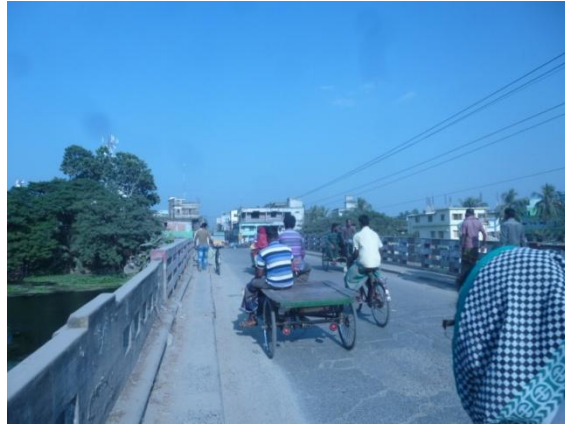
Photograph 4.2: The Bridge over the Kobadak at Jhikargacha.
