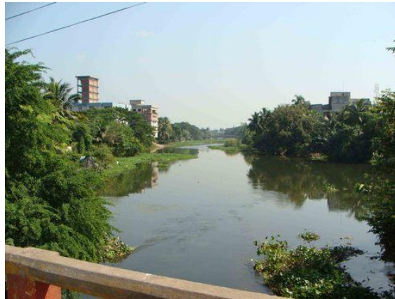
Photograph 4.1: The Daratana Bridge over the Mukteswari River at Jessore Sadar and encroachments from both ends of the river.
