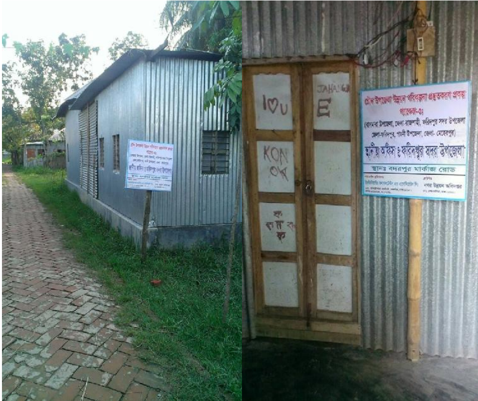
Photo 4-2: Hired Local project Office at Faridpur Sadar Upazila.
