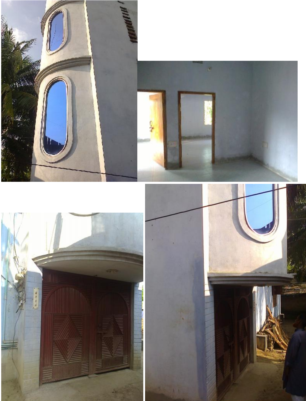
Photo 4-3: Hired Local project Office at Gangni Upazila.
