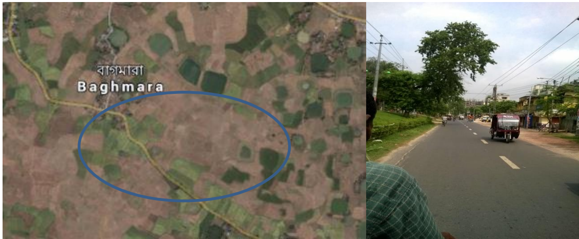
Photo 3-36: Bagmara road (Source: Field Visit, 2015)
