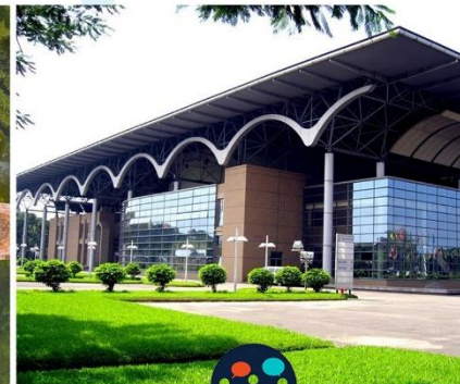
4 Bangabandhu International Conference Center
