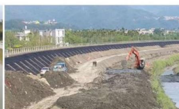
Picture-20.2: Geo Web Embankment
