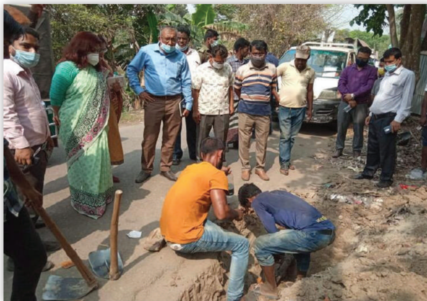
A view of eviction operation of illegal gas distribution line
