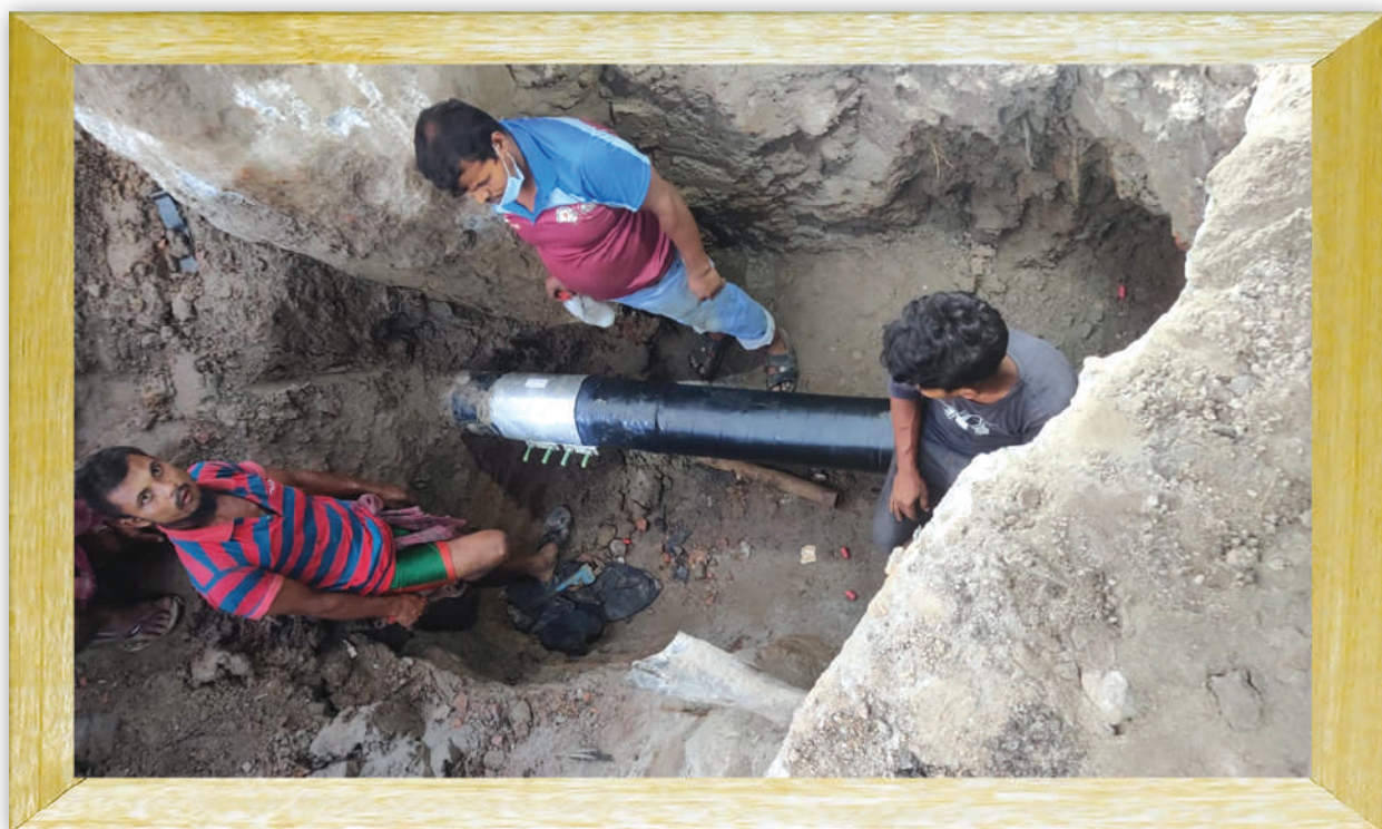
Repiering of Gas Pipeline
