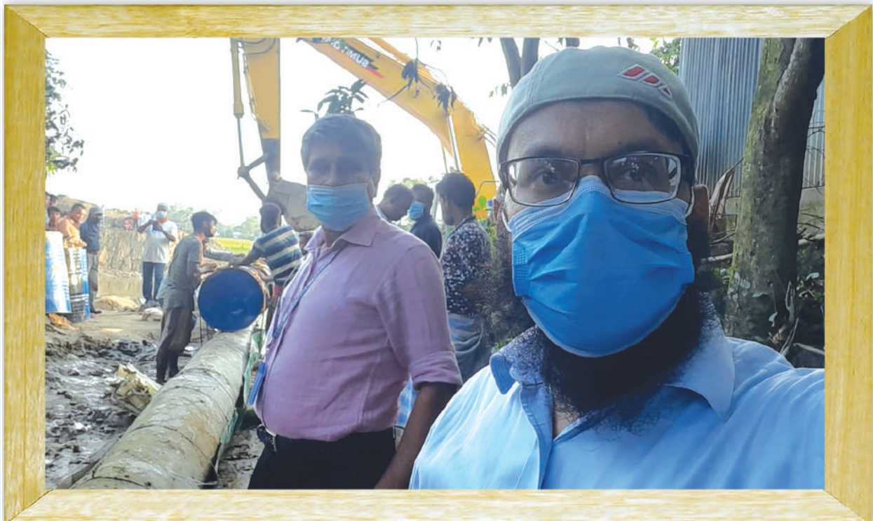
A view of on Pipeline Construction Activities
