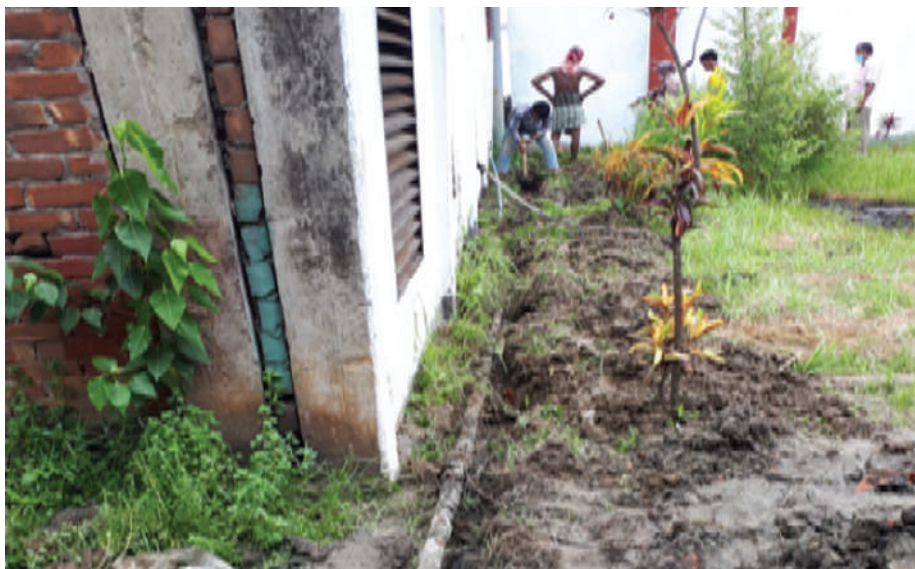
Disconnection operation of illegal gas distribution line due to bypass line in industries
