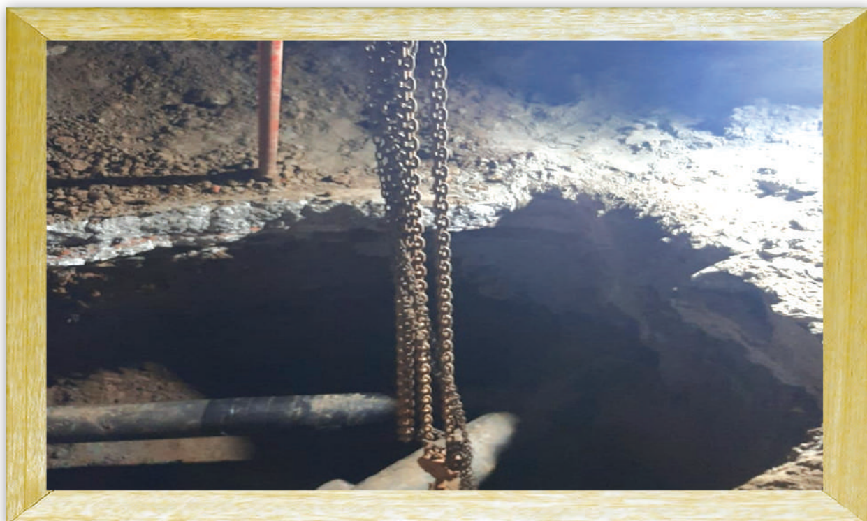
Repiering of Gas Pipeline
