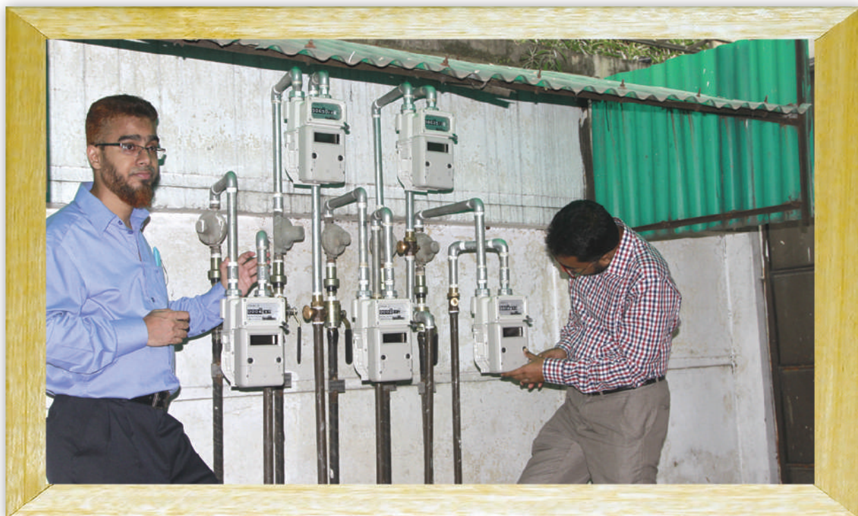
Installation of Prepaid Meter at Titas Franchise Area
