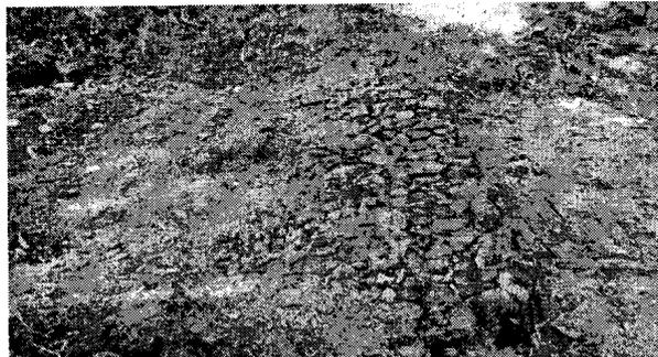
The whole depth of gabion is filled with earth transported from the upper end during the rainy season
