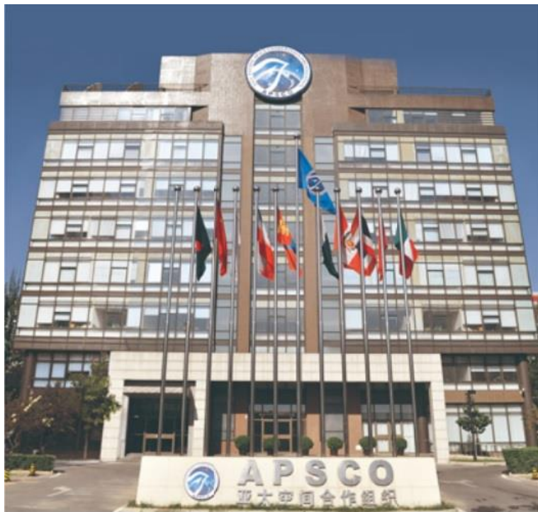
Photograph 7.1: APSCO Headquarters in Beijing (Source: www.apsco.int )
