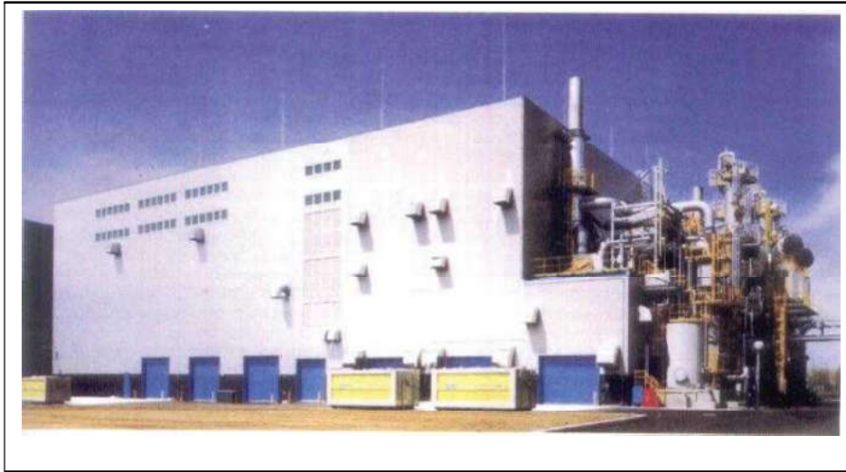
Fig. 20: Waste Plastics to Oil Production Facility in Japan
