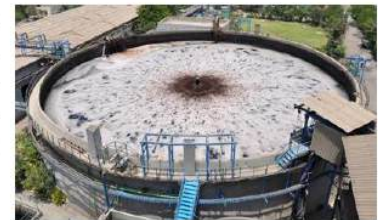
Fig. 8 Anaerobic digestion
