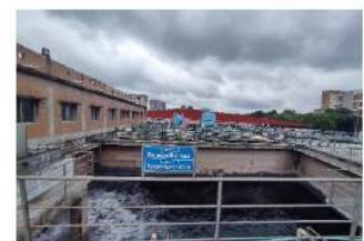
Fig. 6 Equalization tank
