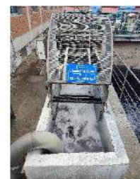
Fig. 5 Automatic rotary bar
