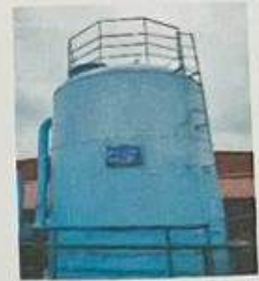
Fig. 21 Multigrade filter
