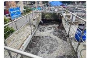
Fig. 11 Distribution tank
