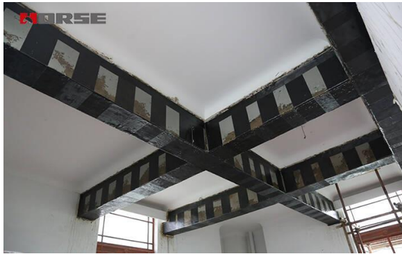
Figure 02: Beam with U-shaped CFRP sheet
