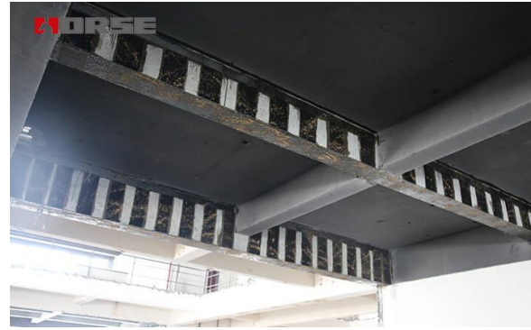
Figure 03: Beam with Side-bonded CFRP sheet
