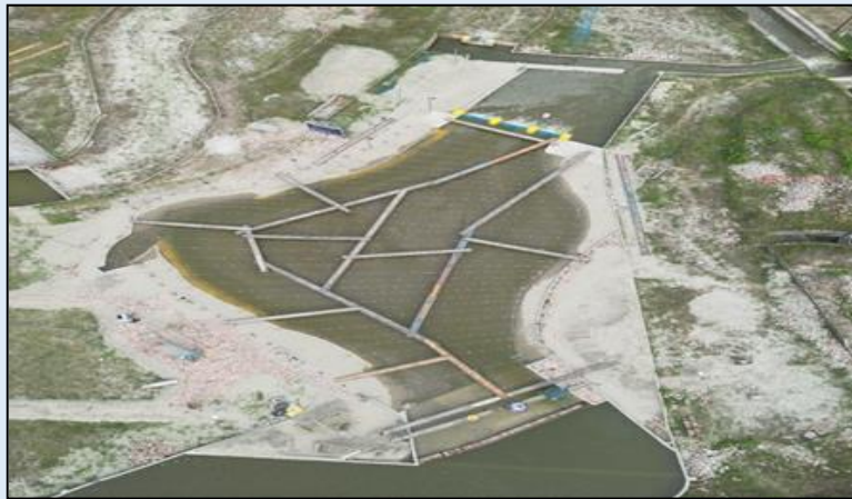
Figure: A view of Physical Model Study of Surface Water Treatment Plant for Rajshahi WASA.
