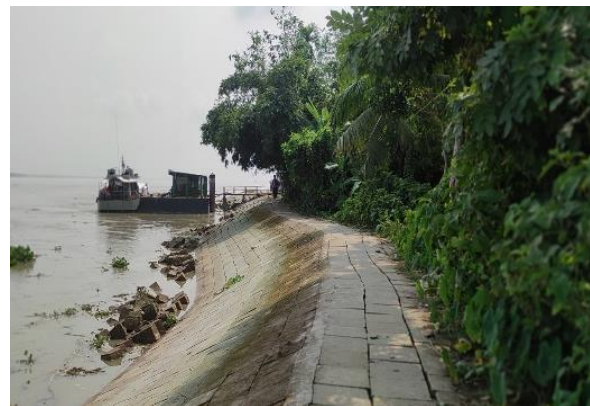
Fig. 3. Existing hard material protection (CC block) works at Dighirpar Launch Terminal.
