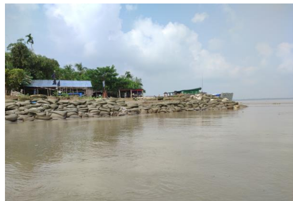
Fig. 4. Existing geobag protection works in the upstream of Dighirpar Launch Terminal.
