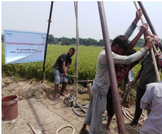
Figure-4: Showing the Soil Boring Works
