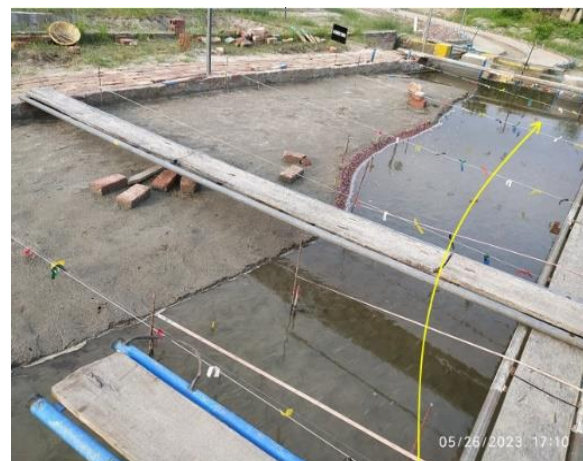
Fig. 8. Bank erosion occurred at the left bank of Brahmaputra model under base condition (T1 100yr ).
