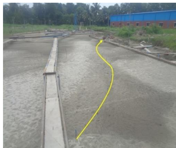
Fig. 19. Alignment of silted dredged channel.
