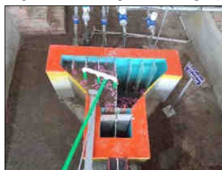
Fig. 9. Backwashing process of fine screen chamber and pipe
