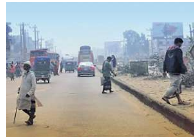
FIGURE 2.3 Section of N3 lacking safe crossing and walking facilities for pedestrians
