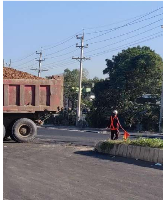
Equipped flagman at under construction zone
