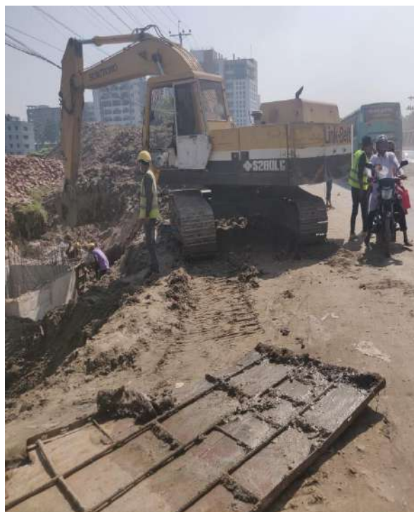
Risky edge drop of road side at Airport to Jaydevpur Under-construction zone
