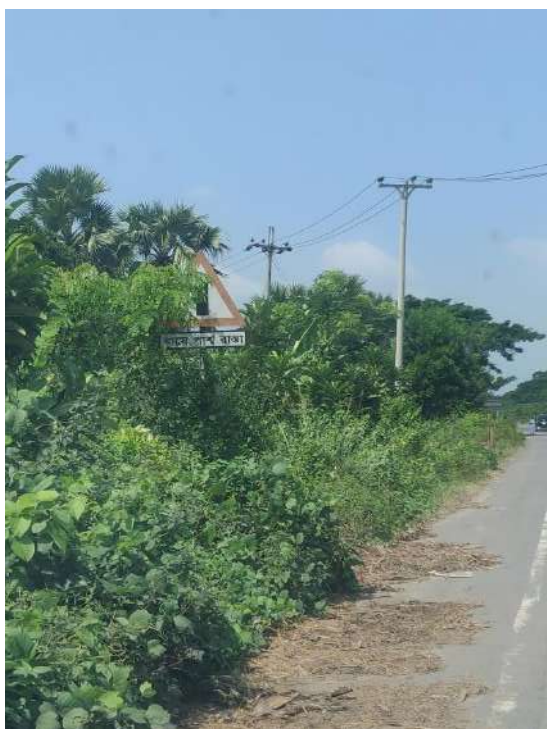
Road side bush occupying earthen shoulder at Ch.+ 98 to Ch.+101
