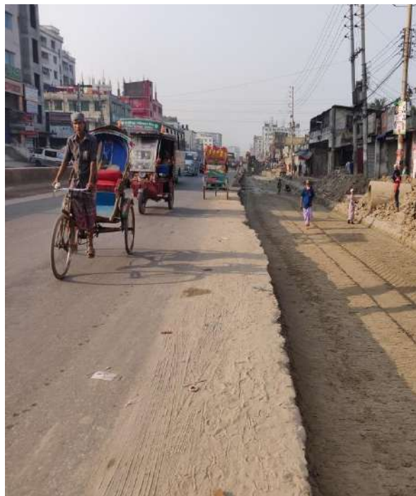
Risky edge drop of road side at Airport to Jaydevpur Under-construction zone
