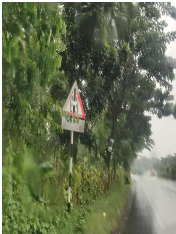
Less visible road sign at Ch.+148 to Ch.+156
