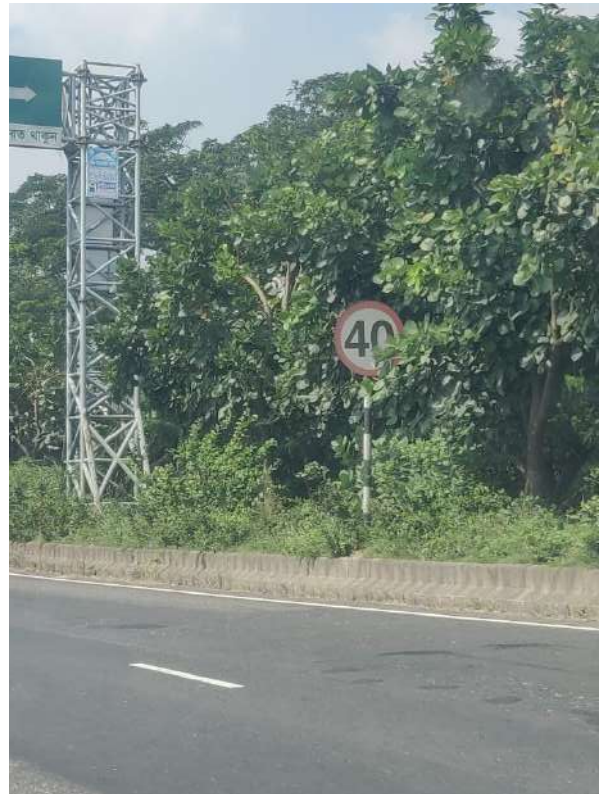
Disturbed road sign visibility issue within Ch.+55 to Ch.+56
