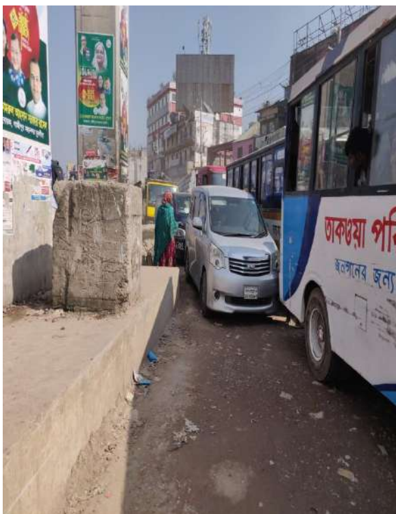
Encroached road at Airport to Jaydevpur Under-construction zone
