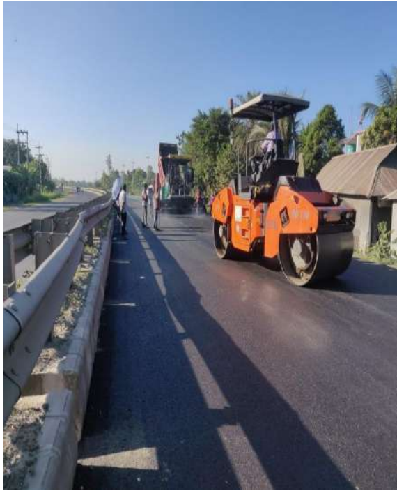
Site Inspection at under construction zone
