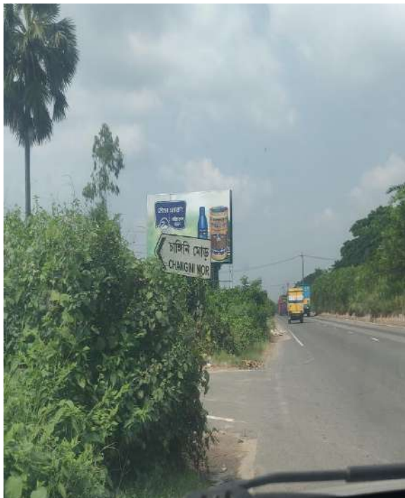
Disturbed road sign at Ch.+88 to Ch.+92
