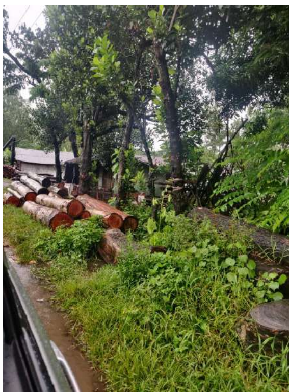
Road side occupancy in shoulder within Ch.+160 to Ch.+166
