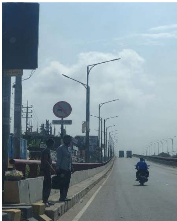
Risky pedestrian standing on meadin at Ch.+ 110 to Ch.+116
