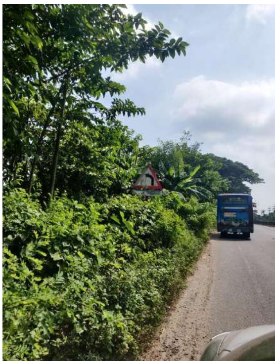
Less visible road sign at Ch.+141 to Ch.+144
