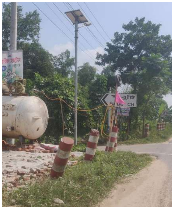
Inadequate shoulder within Ch.+110 to Ch.+112
