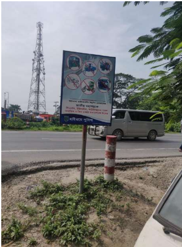
Risky edge drop and structure within Ch.+53 to Ch.+54
