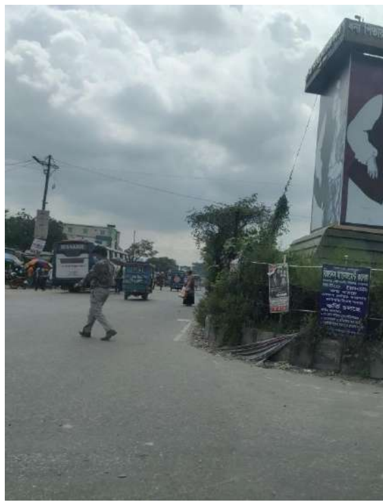
Risky median with no reflectivity at Ch.+ 5 to Ch.+6
