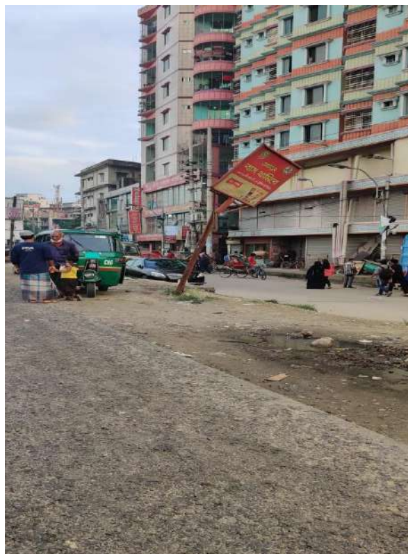
Disturbed road sign within Ch.+ 2 to Ch.+4
