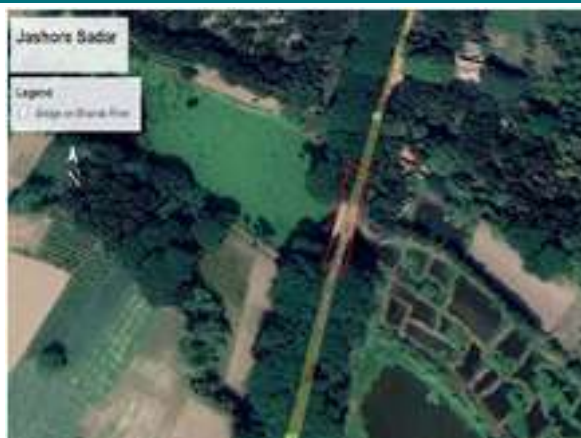
Bridge over Bhairab River, Contract- 3:
