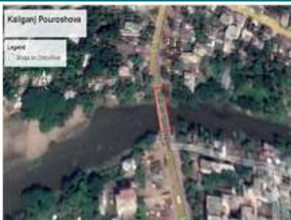
Bridge over Chitra River, Contract- 2
