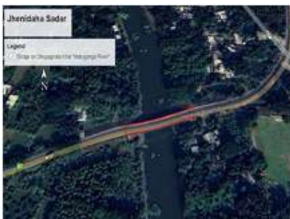
Bridge Over Naboganga River, Contract- 1
