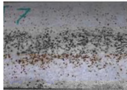
Photo18-2 Surface area of 20~30 rusting
