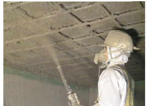
Spraying repair mortar
