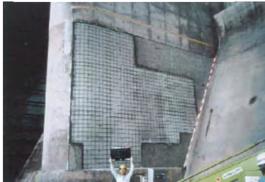
Cleaning of Concrete and Rebar
