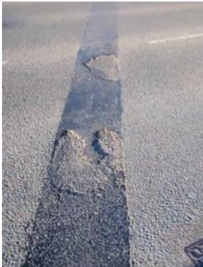
Damaged Asphaltic plug joint
