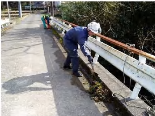
Fig. 2-1 Removing of soil and weed by shovel Fig.2-2 Removing of soil and weed by jet water
