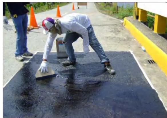
Photo 17-2 Asphalt Compound Method
