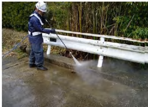
Fig. 2-1 Removing of soil and weed by shovel Fig.2-2 Removing of soil and weed by jet water
