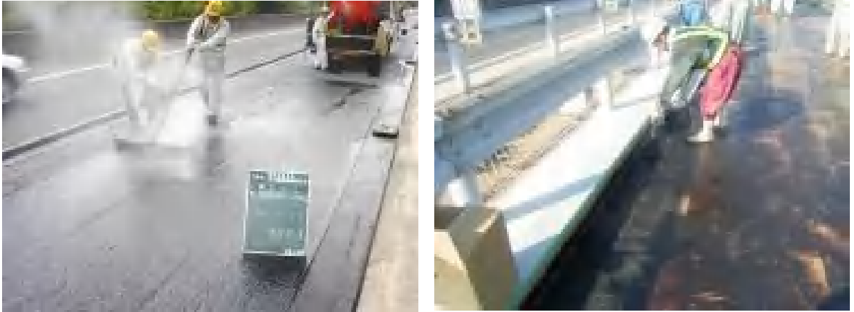
Figure 4-17 Waterproofing of deck slab (Asphalt compound type)
