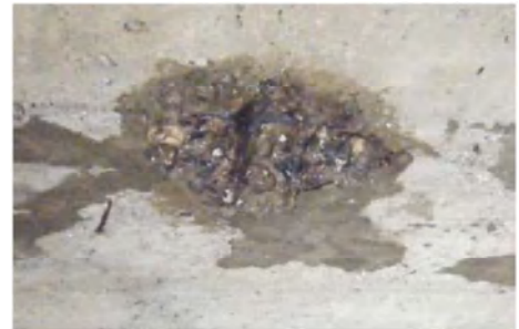
Epoxy bonding coat
