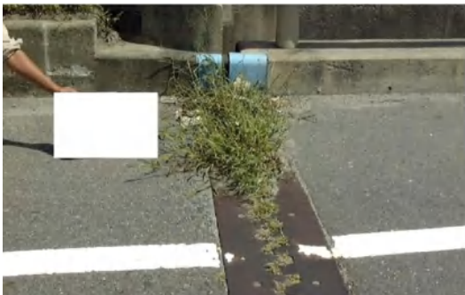
Fig.2-7 Blocked expansion joint
