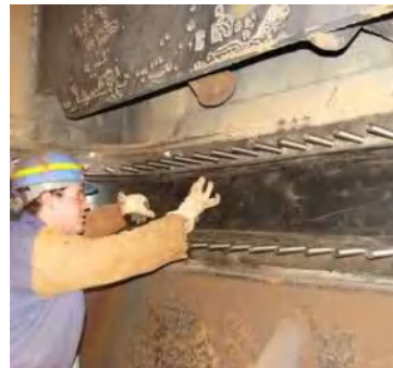
Fig.2-8 Cleaned expansion joint tube
