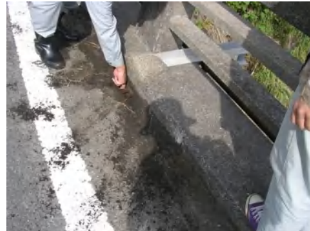
Fig.2-4 Removing the soil by brush
