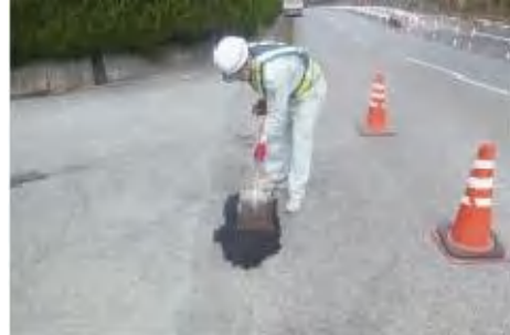
Photo5-3 Patching of Repair Material
