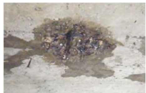
Epoxy bonding coat
