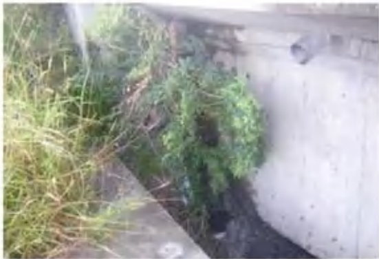
Photo 1-1-7 Vegetation on substructure
