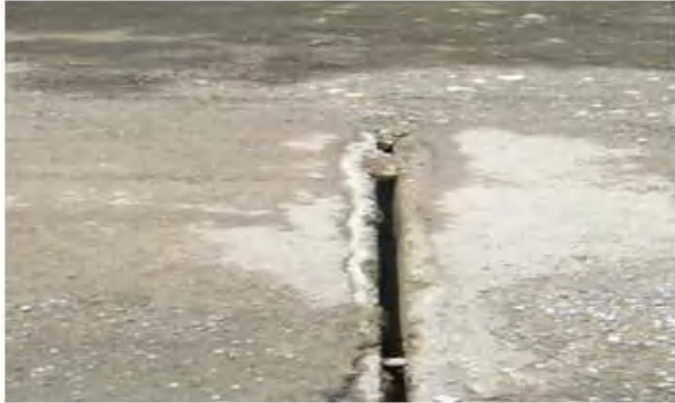
Photo 1-1-6 Debris on bearing
