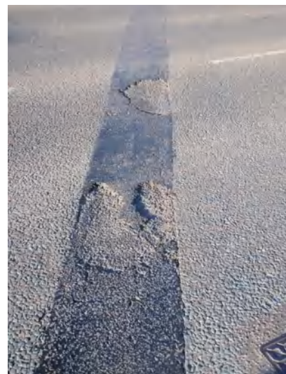
Figure 4-6 Asphaltic plug joint (left) and its surface damage (right)
