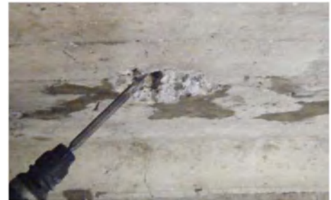
Removal of defect concrete
