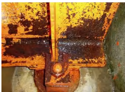
Fig.2-12 Cleaned steel plate by jet water
