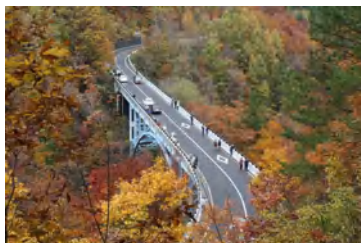
Fig.2-19 Tree growth under the bridge
