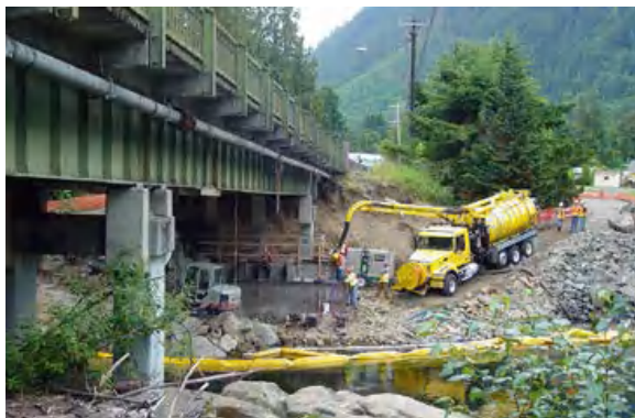
Figure 4-12 Scour repair work by special heavy equipment
