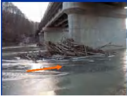
Fig. 2-14 Pier with flow obstruction
