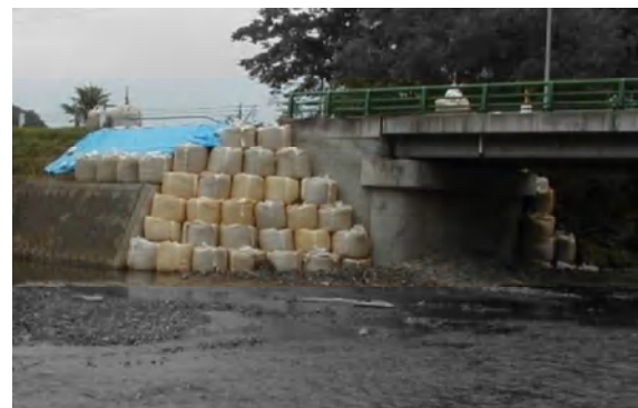
Photo 3-14-4 Placing Sand Bags
