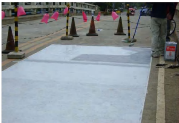
Photo 17-1 Rubberized Membrane Method
