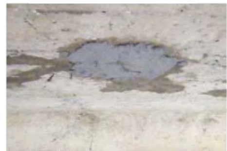
Curing after Patching
