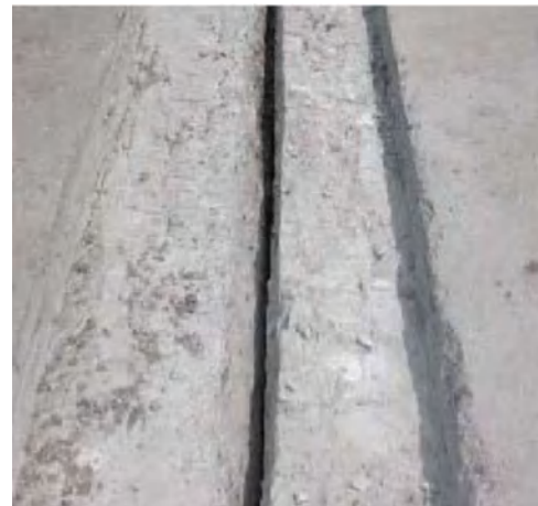
After removing Sealant of Asphaltic plug joint
