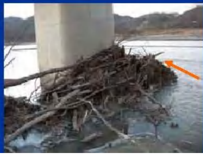
Fig.2-15 Pier with flow obstruction
