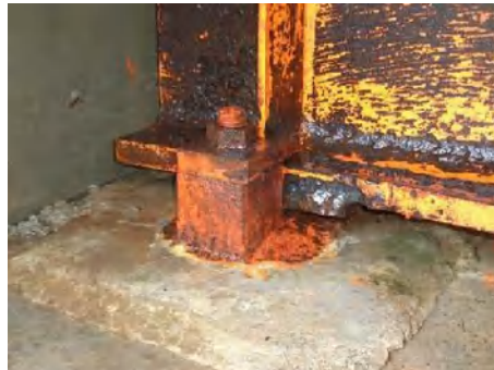
Fig.2-11 Cleaned Bearing by jet water
