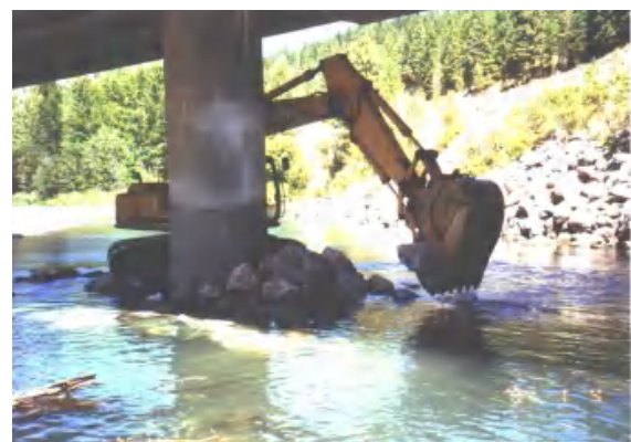
Placing Special Heavy Loose Rip Rap
