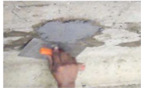
Filling up in Patching
