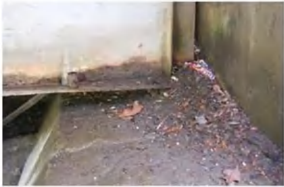
Photo 1-1-6 Debris on bearing
