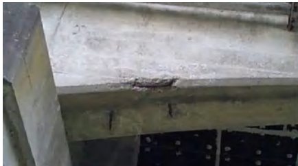
Fig.2-23 exposed Rebars (small area) Fig.2-24 Treatment of exposed rebar by brush
