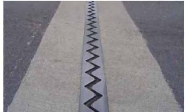
Figure 4-8 Steel Expansion Joint
