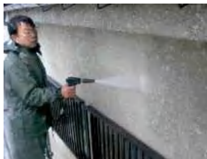
Fig.2-13 Cleaning concrete surface by jet water
