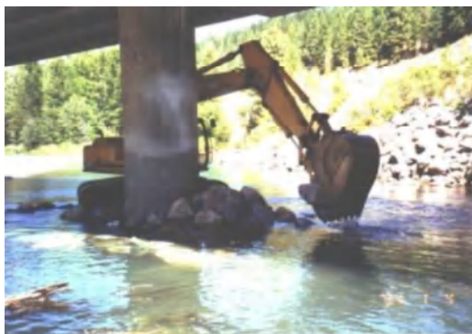
Placing Special Heavy Loose Rip Rap
