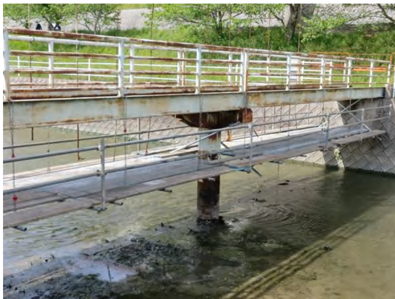
For example of Scaffold
