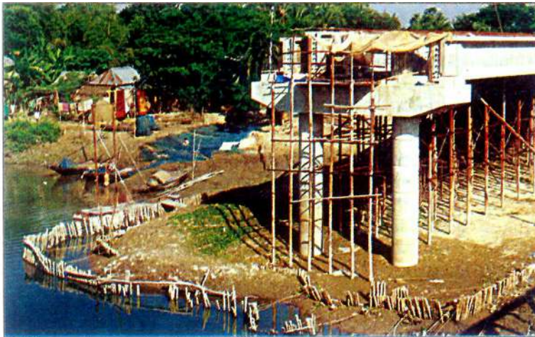
Bridge under construction near Bhanga.
