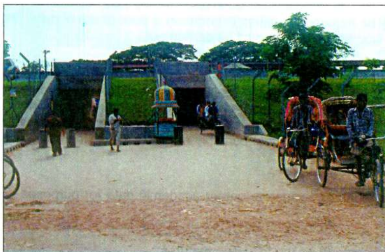
Rickshaw and pedestrian underpass, Bhairab.
