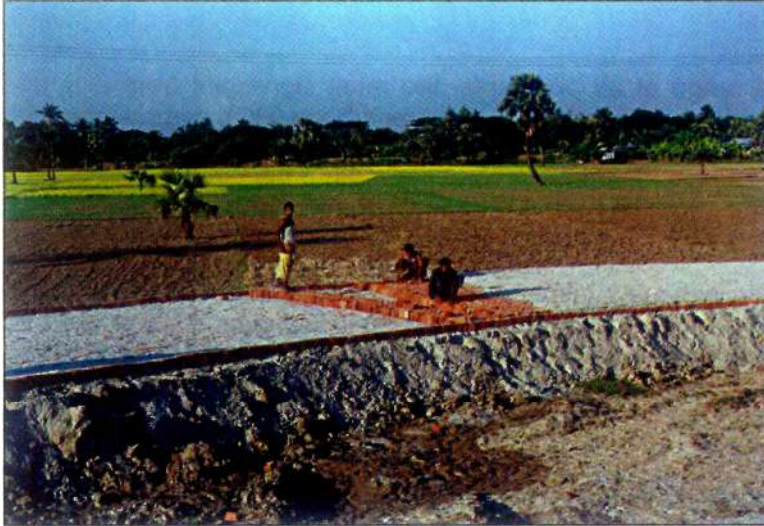
Temporary diversion works.
