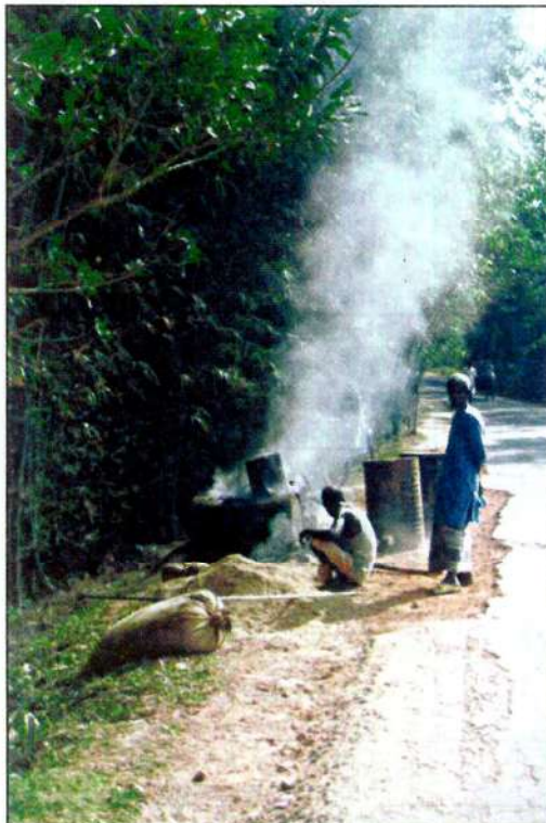
Heating tar for road repairs.
