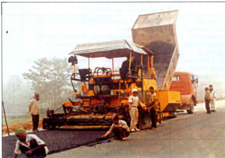
Road pavement construction.
