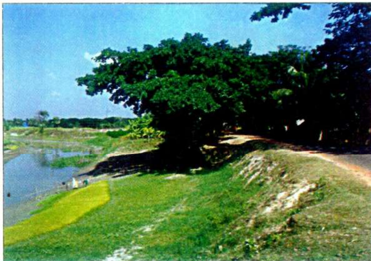
Trees help protect embankments from erosion.
