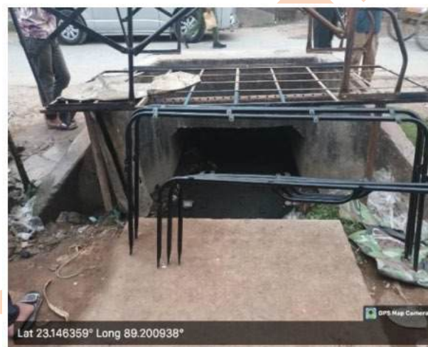
Exhibit 3-1: Existing Culverts along the Project Corridor
