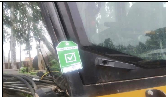
Image 22: Implemented Green tag at the construction area
