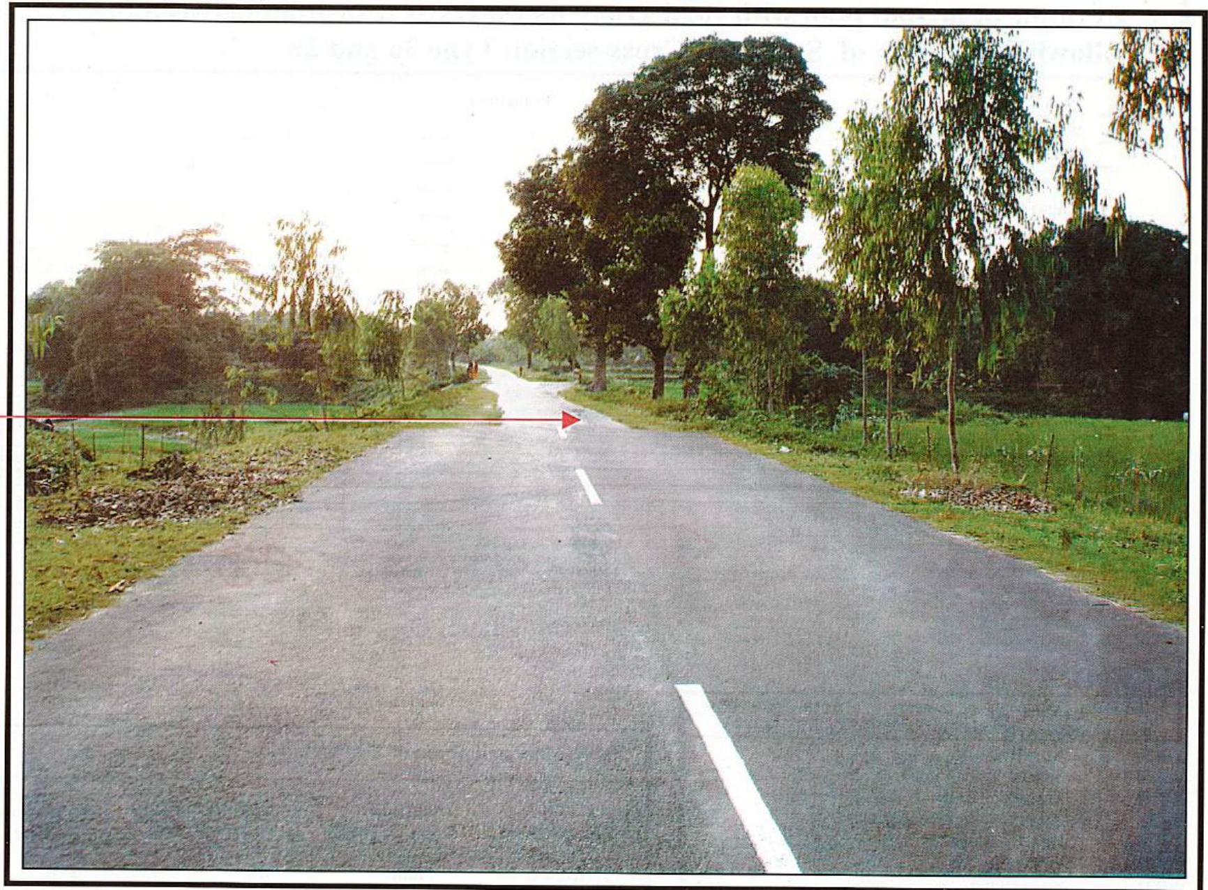
Photo from Dinajpur - Thakurgaon - Panchagarh National Highway
