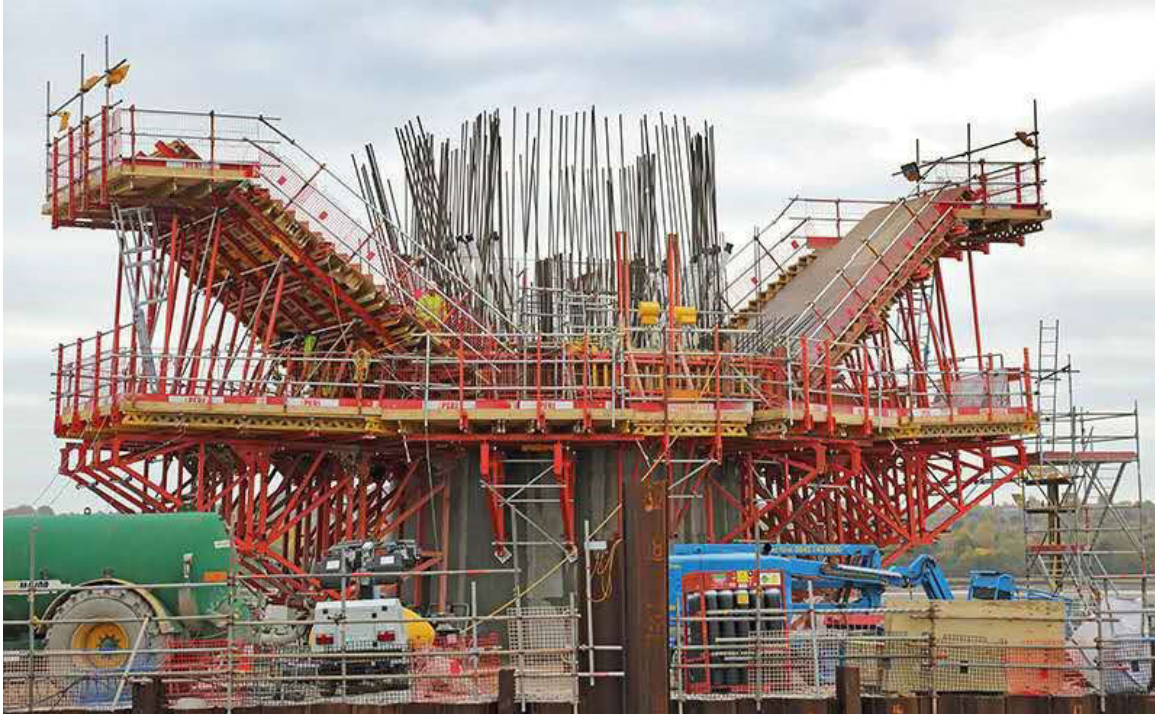
Figure: Example of the safe Working Platform
