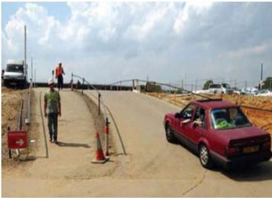
Figure: Pedestrians are segregated from vehicles on this slope
