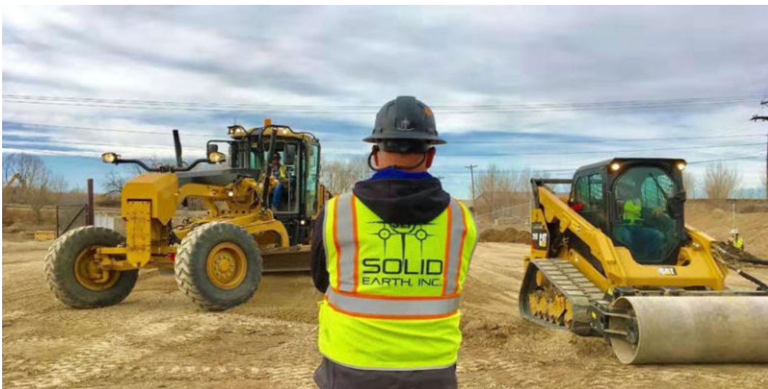
Figure: Safe Embankment work
