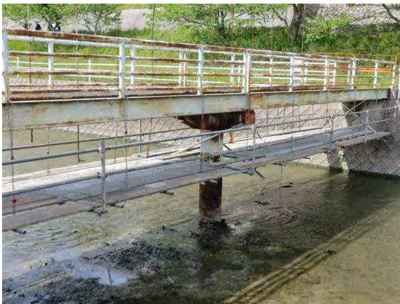
For example of Scaffold
