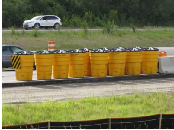
Figure 7.30-1: Inertial sand barrel attenuators.
