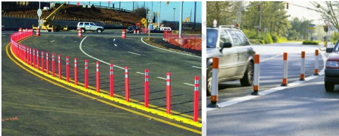
Figure 7.9-2: Typical Lane delineator post.
