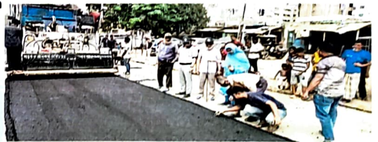
Laying of plastic bituminous layer
