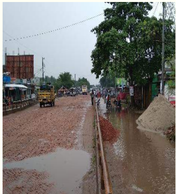
Pavement without DBS within Ch.+ 118 to Ch.+120
