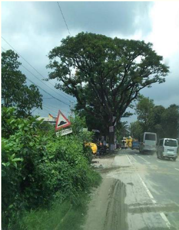
Disturbed road sign within Ch.+26 to Ch.+28 is misplaced and less visible
