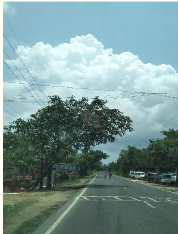
Below standard zebra crossing without speed calming arrangement within Ch.+ 335 to Ch.+337
