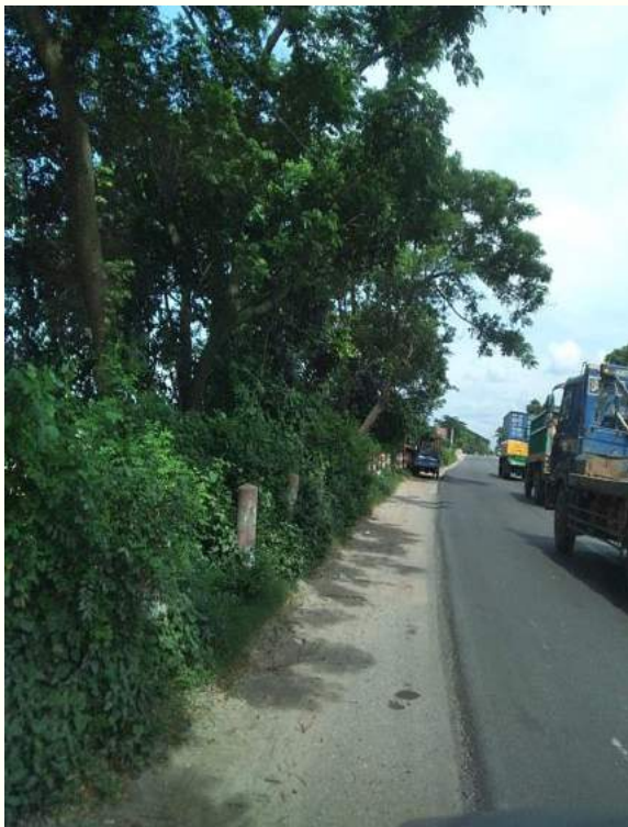
Invisible roadside posts Ch.+ 15 to Ch.+17
