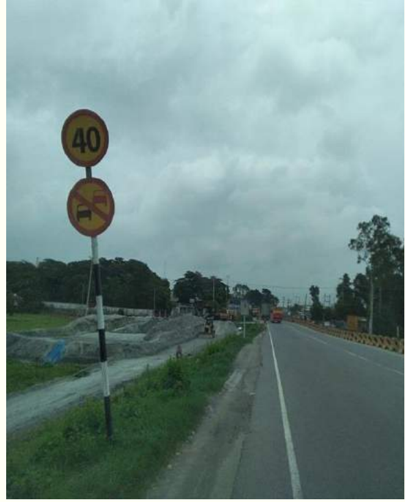
Wrongly colored road sign within Ch.+35 to Ch.+37
