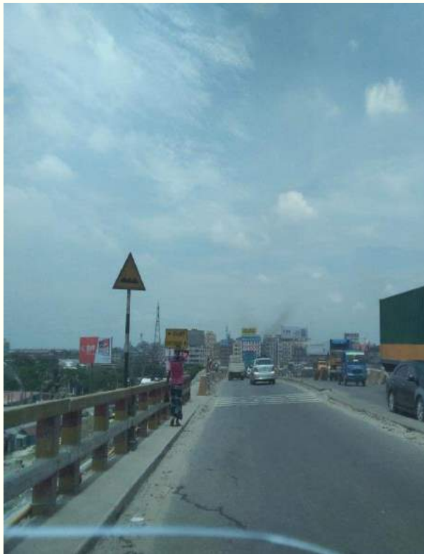
Improper bridge facilities within Ch.+7 to Ch.+9
