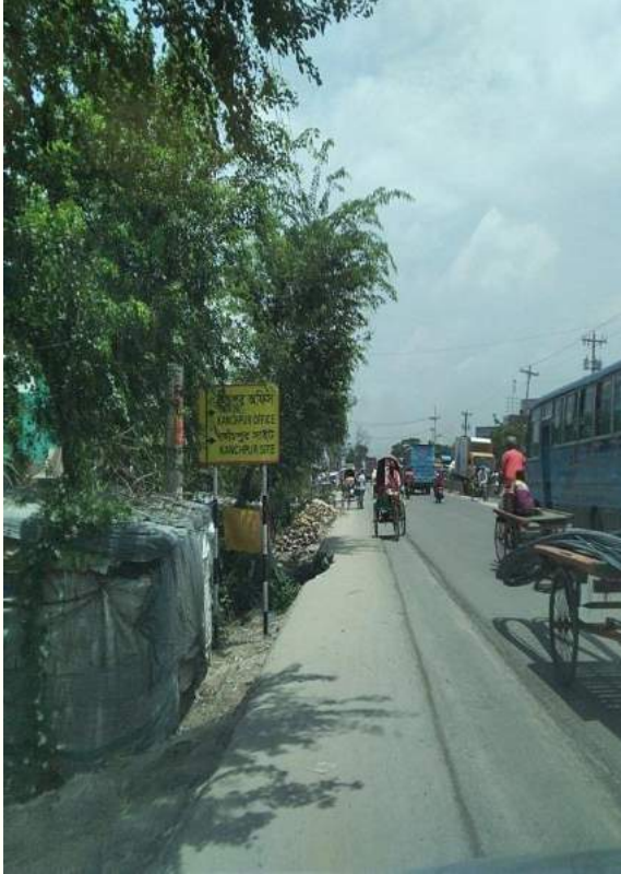
Risky drop and poor sign visibility within Ch.+ 9 to Ch.+11
