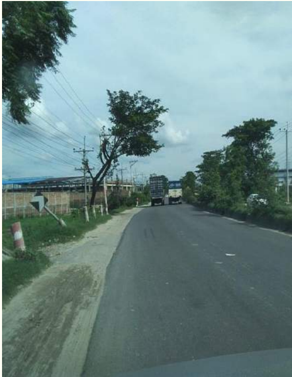
Disturbed sign within Ch.+17 to Ch.+19
