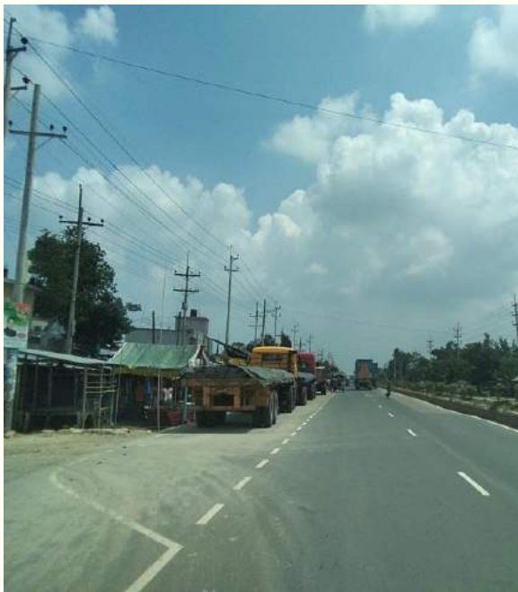
Bus bay occupied by heavy loaded trucks within Ch.+63.6 to Ch.+65.6
