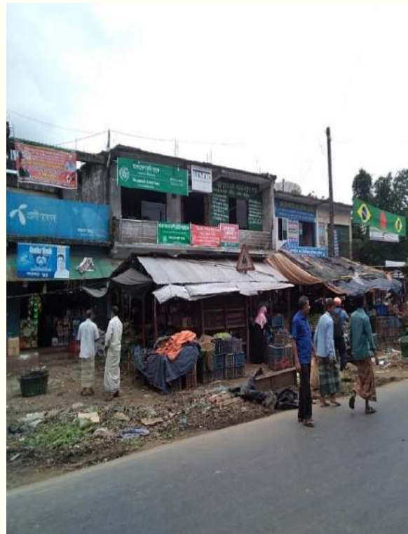
Roadside business in shoulder within Ch.+321 to Ch.+323
