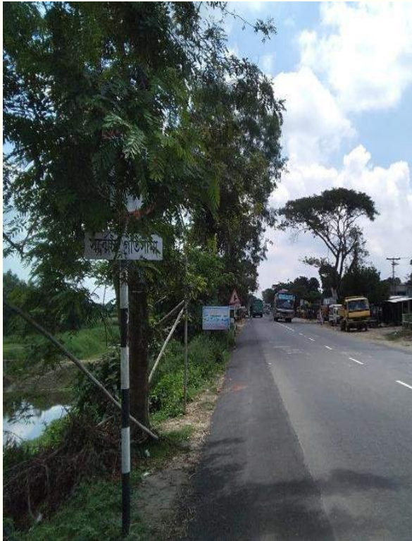
Less visible road sign within Ch.+60 to Ch.+62
