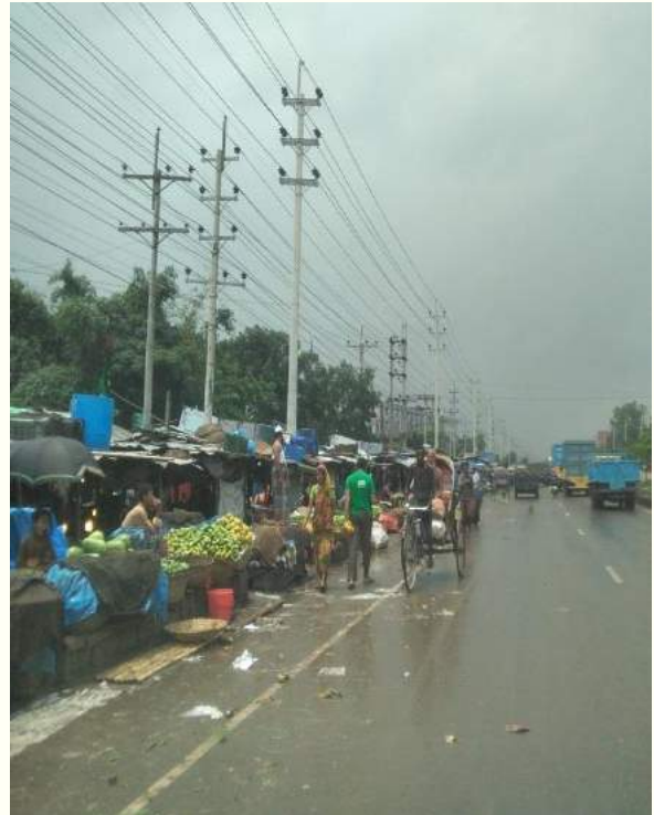
Illegal roadside activity within Ch.+49.8 to Ch.+51.6
