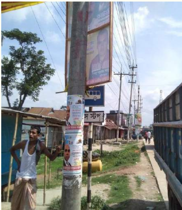
Improper placement of sign within Ch.+93.5 to Ch.+95.5
