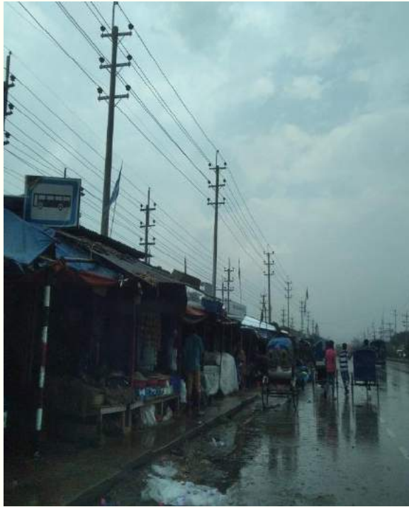
Unauthorized roadside business within Ch.+51.6 to Ch.+53.6
