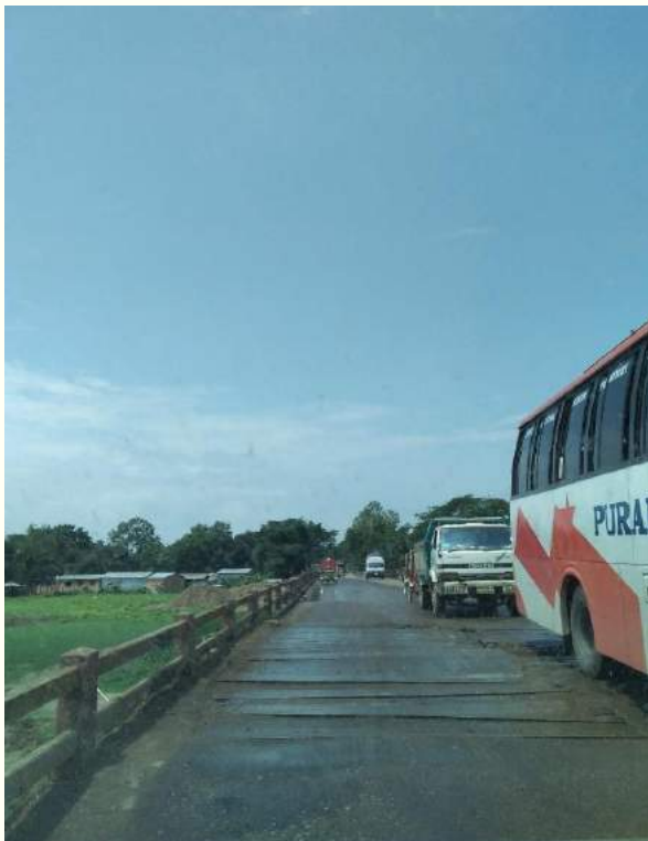
Bridge having no footpath and delineation at Ch.+ 331 to Ch.+333
