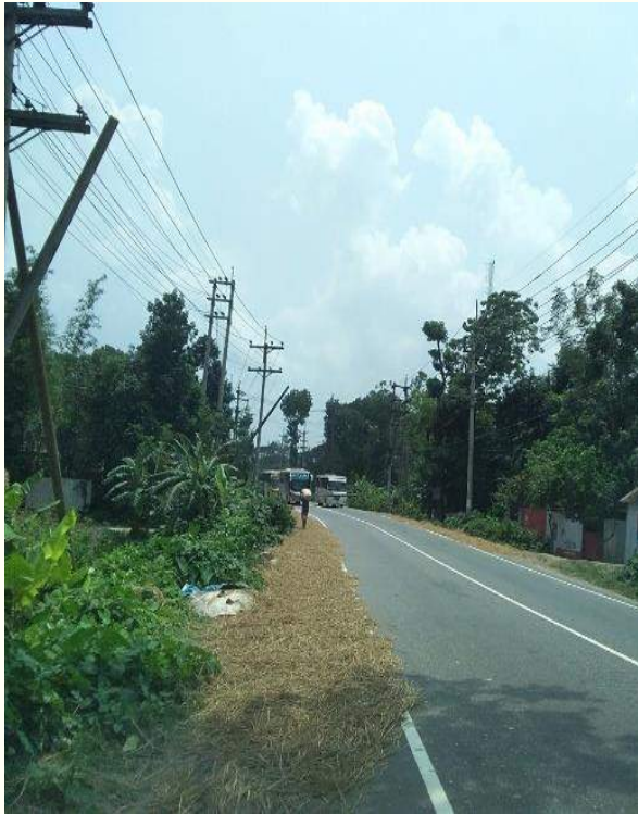
Unauthorized roadside business within Ch.+48 to Ch.+50
