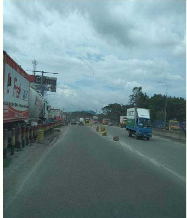
Hazardous median blocks within Ch.+23 to Ch.+25
