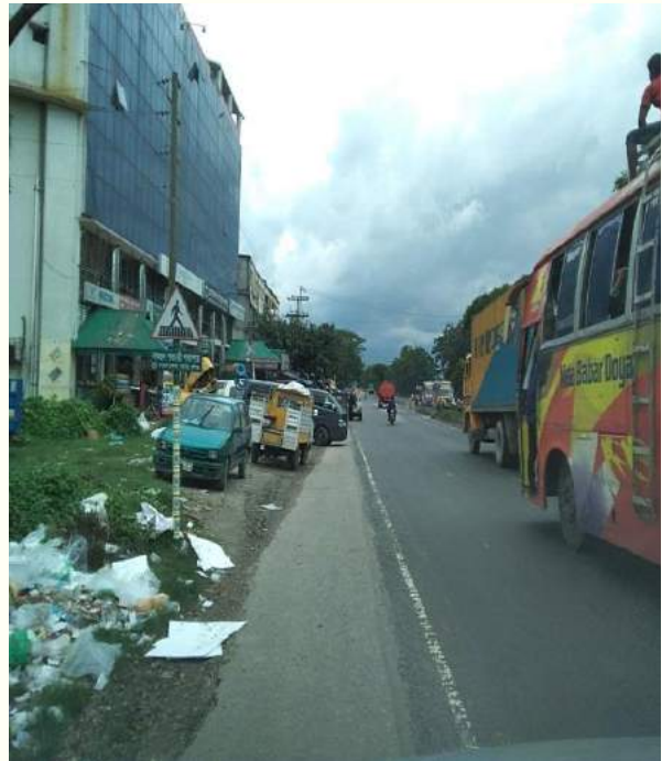
Wrongly designed road sign within Ch.+29 to Ch.+31
