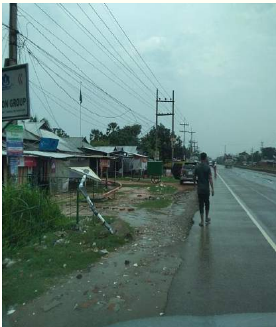
Disturbed & broken sign within Ch.+57.6to Ch.+59.6
