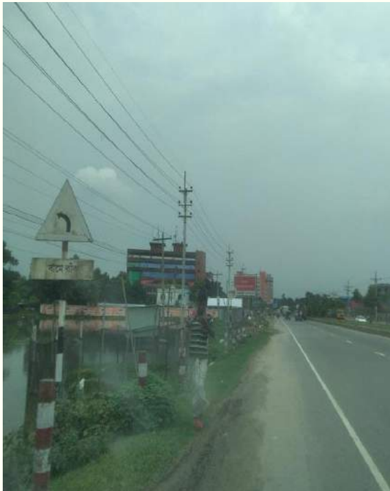
Faded road sign within Ch.+39.8to Ch.+41.8
