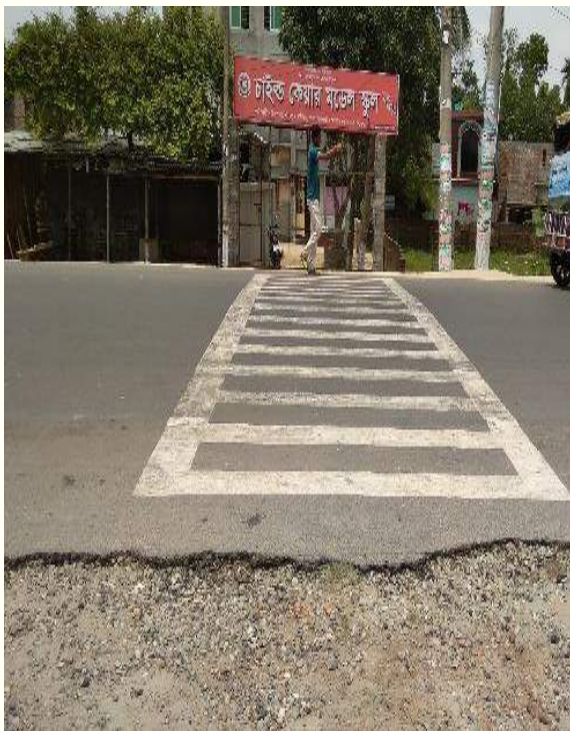
Unauthorized zebra crossing without traffic calming device within Ch.+ 138 to Ch.+140
