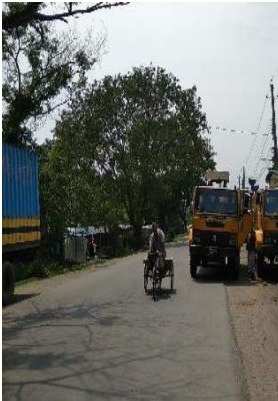
Unauthorized parking within Ch.+ 98 to Ch.+100
