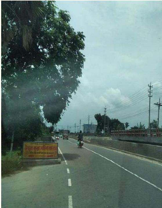
Unauthorized hazardous roadside structure within Ch+101.5 to Ch+103.5
