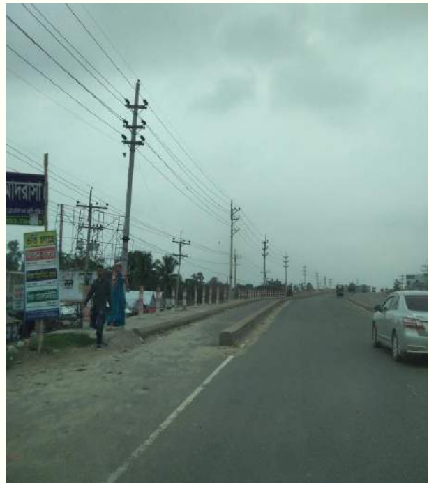
Divider without warning sign at Ch.+23.8 to Ch.+25.8
