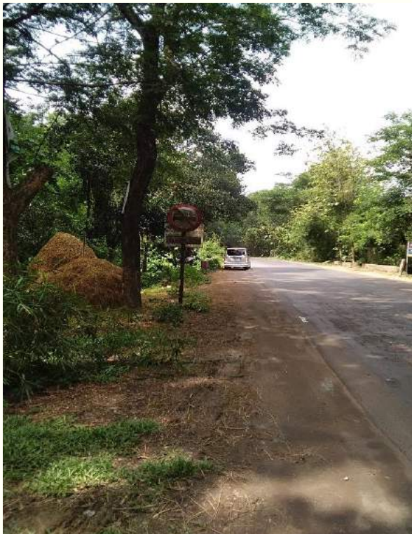
Less visible road sign at Ch.+311 to Ch.+313
