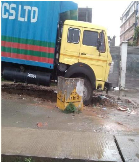
Hazardous km post installed on roadside area within Ch.+25.8 to Ch.+27.8
