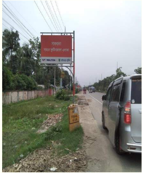
Risky km post and unknown sign post in earthen shoulder within Ch.+21.8 to Ch.+23.8
