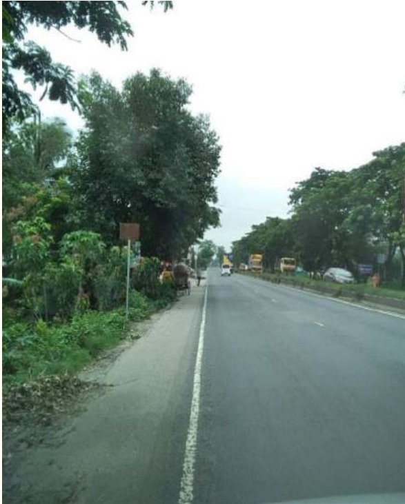
Damaged road sign within Ch.+33 to Ch.+35
