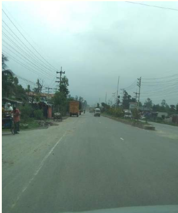
Poor road marking within Ch.+27.8 to Ch.+29.8
