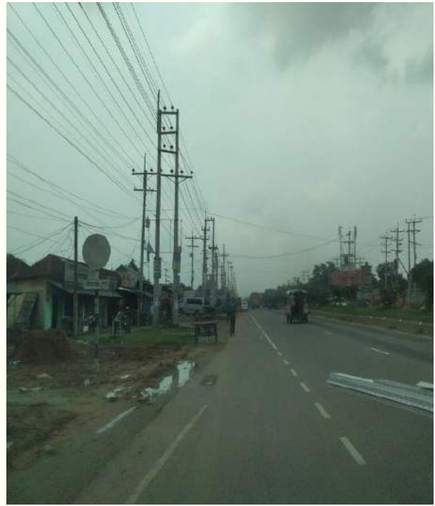
Faded road sign within Ch.+43.8 to Ch.+45.8
