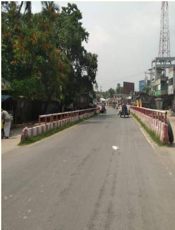
No marking and sign at barrier within Ch.16 to Ch.+18
