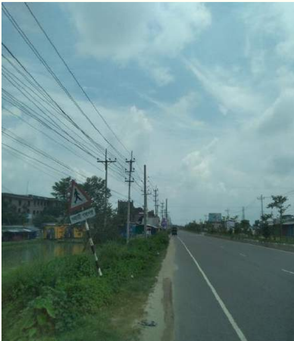
Disturbed sign post within Ch.+99.5to Ch.+101.5
