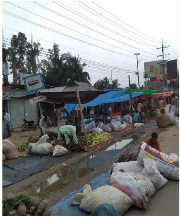
Unauthorized roadside business at Ch.+27.8 to Ch.+29.8
