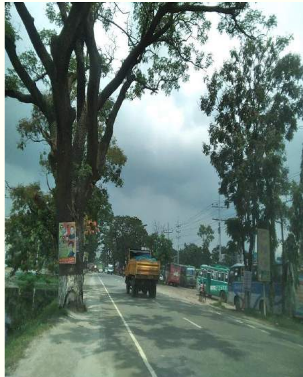
Earthen shoulder within Ch.+26 to Ch.+28 gets blocked by roadside large tree
