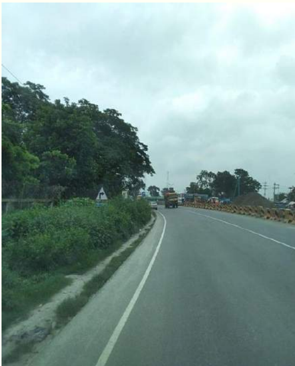
Improper placement of sign within Ch.+35 to Ch.+37
