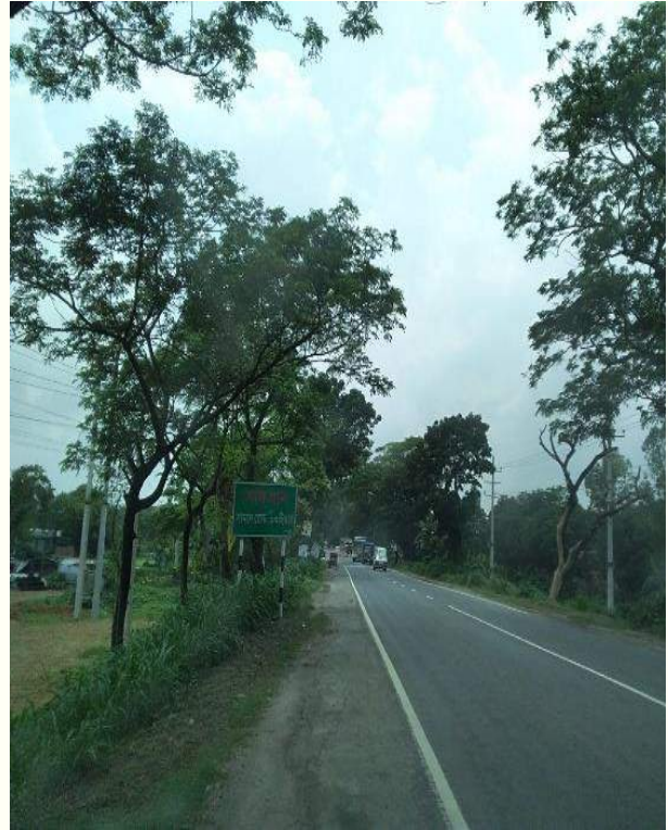
Sign post on earthen shoulder within Ch.+34 to Ch.+36 causing risk
