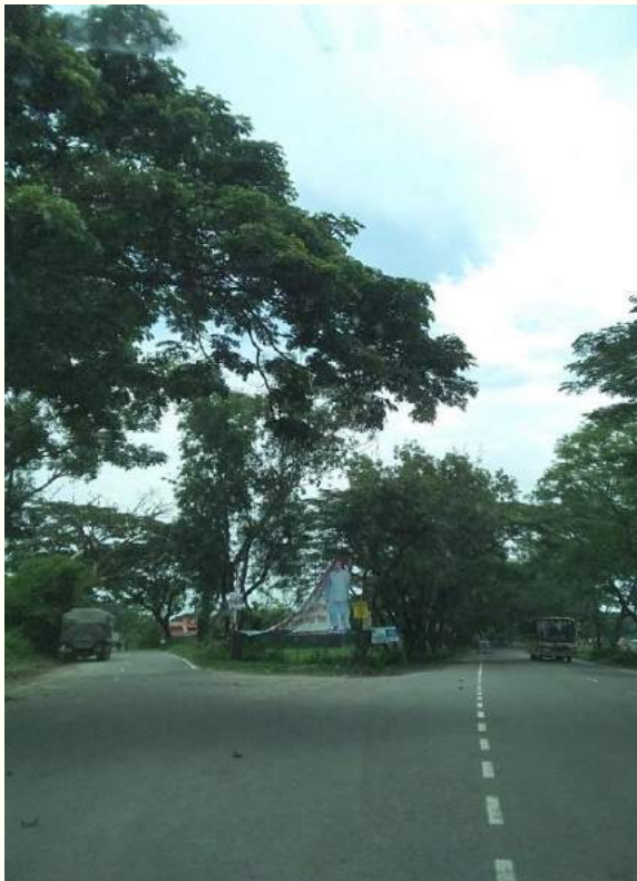
Y-intersection without warning sign within Ch.+255 to Ch.+257 causing high risk
