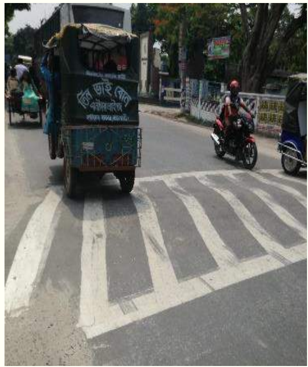
Wrong designed raised pedestrian crossing within Ch.+140 to Ch.+142
