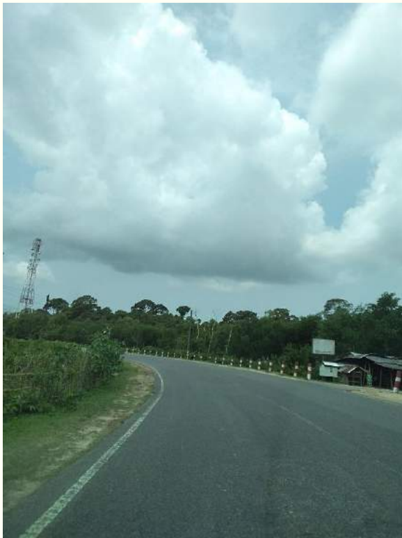
Curve section without chevron sign at Ch.+369 to Ch.+371
