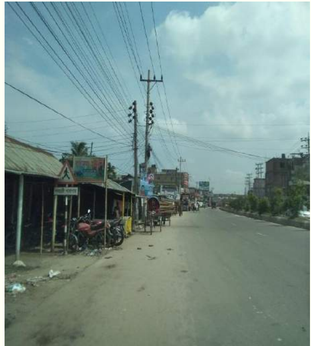
Improper placement of sign & unauthorized occupancy within Ch.+89.5 to Ch.+91.5
