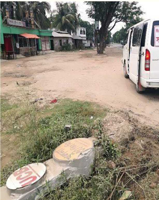
Unknown and disturbed km sign post within Ch.+84 to Ch.+86
