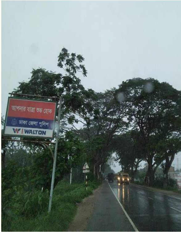
Risky concrete pole in earthen shoulder within Ch.+26 to Ch.+28
