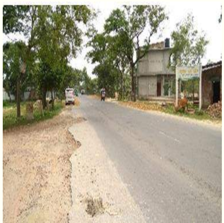
Wrongly colored road sign within Ch.+35 to Ch.+37
