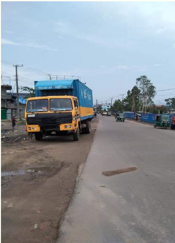
Unauthorized risky parking and shoulder drop within Ch.+ 261 to Ch.+263
