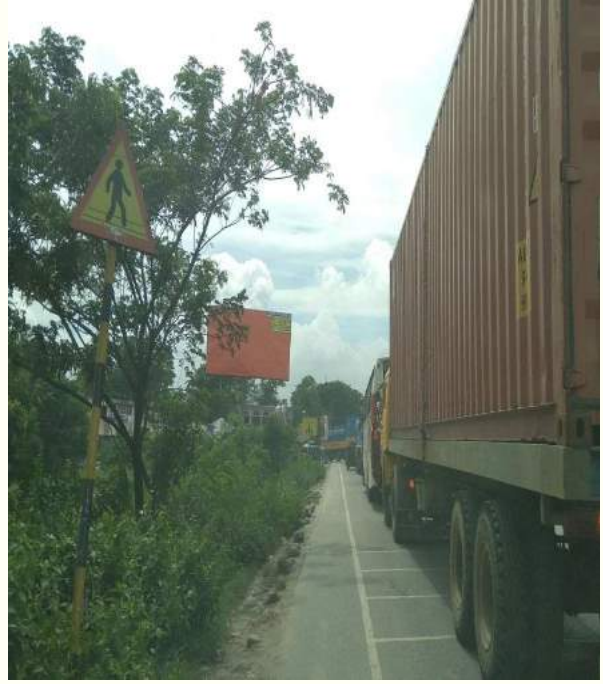
Wrongly designed sign within Ch.+25 to Ch.+27
