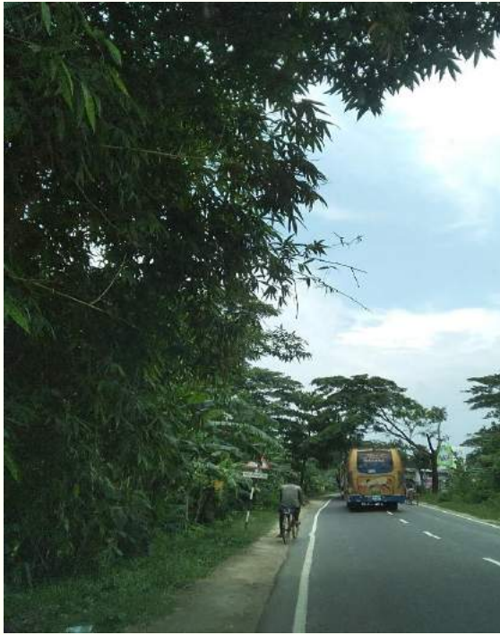
Poor visibility of road sign within Ch.+257 to Ch.+259
