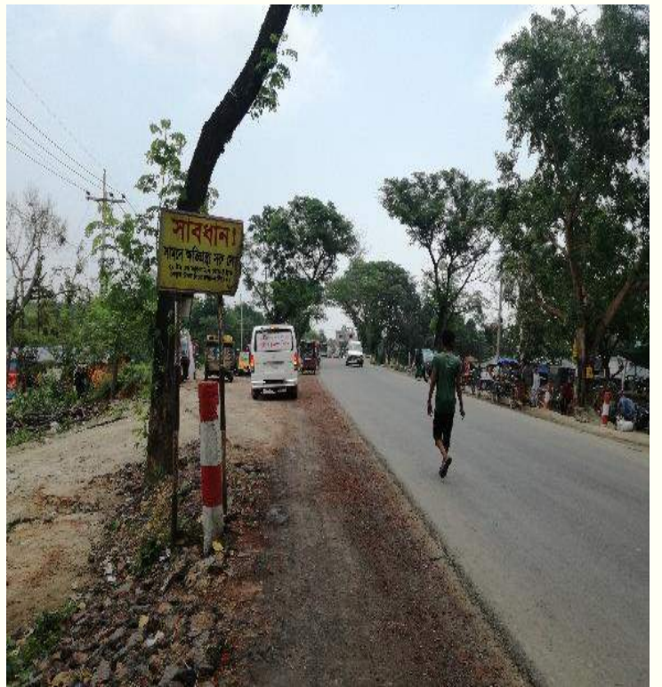
Disturbed sign within Ch.+96 to cjh.+98
