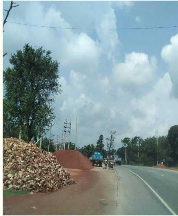
Unauthorized roadside business within Ch.+24 to Ch.+26
