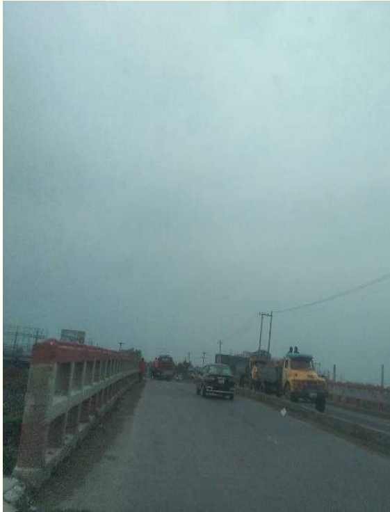
No pedestrian crossing facility on the bridge at Ch.+0 to Ch.+2
