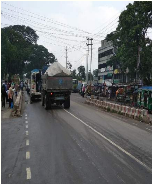
Absence of warning sign at median within Ch.+28 to Ch.+30
