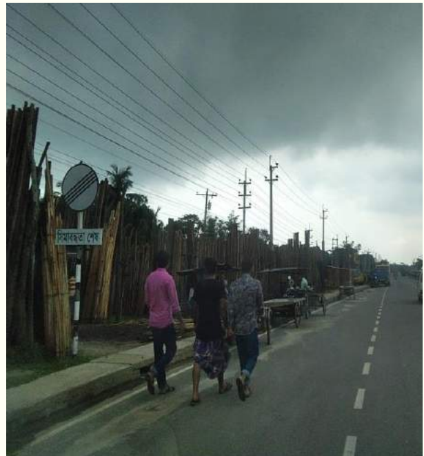
Illegal pedestrian movement within Ch.+59.6 to Ch.+61.6
