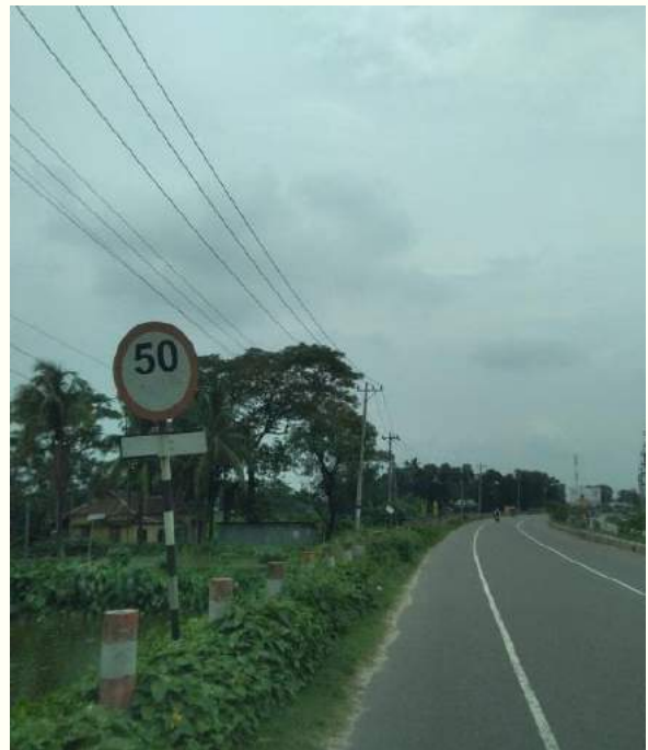
Roadside bushes & wrong marking on curve within Ch.+95.5 to Ch.+97.5
