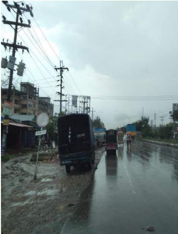
Disturbed road sign and risky shoulder drop within Ch.+23.8 to Ch.+25.8
