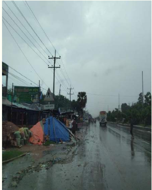
Unauthorized road side business within Ch.+23.8 to Ch.+25.8
