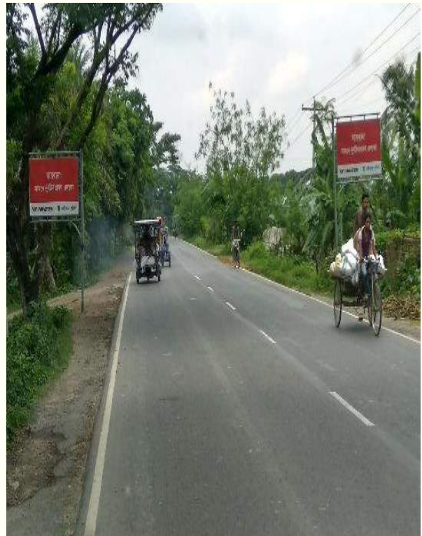
Risky, unknown sign post within clear zone within Ch.+ 72 to Ch.+74
