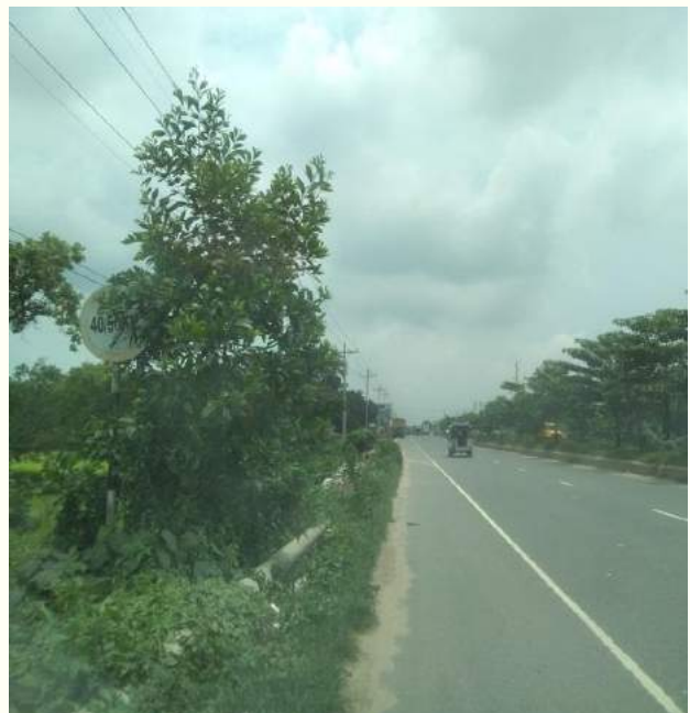
Invisible road sign within Ch.+37.8 to Ch.+39.8
