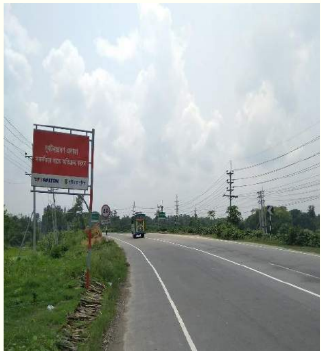
Risky, unknown road sign within Ch.+48 to Ch.+50
