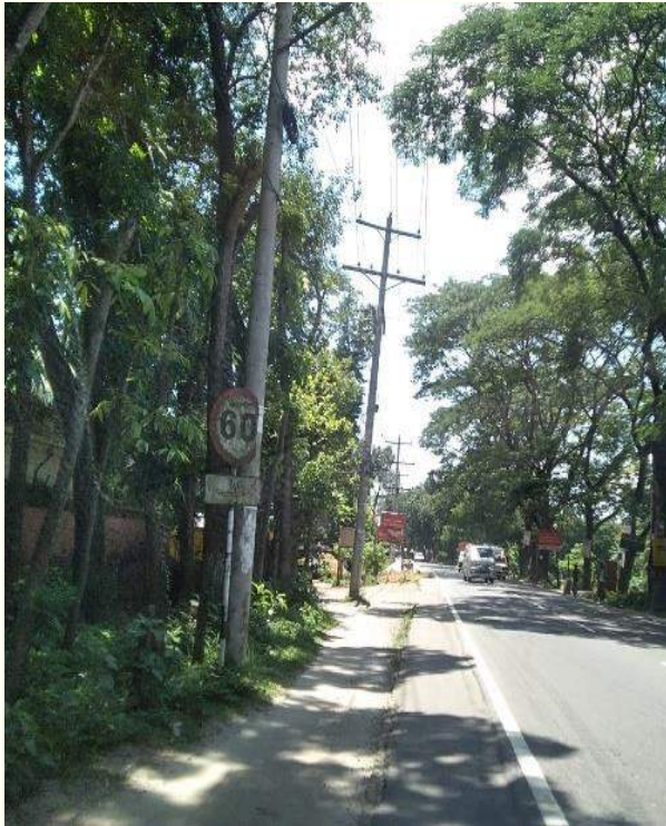
Faded road sign within Ch.+68 to Ch.+70
