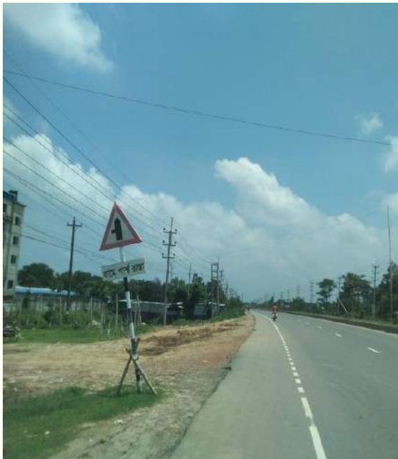
Disturbed sign post within Ch.+71.5 to Ch.+73.5
