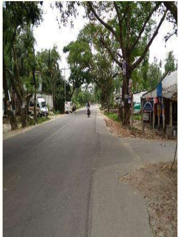
Side road without advanced warning sign within Ch.+106 to Ch.+108
