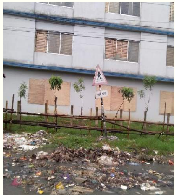
Disturbed and faded road sign within Ch.+21.8 to Ch.+23.8
