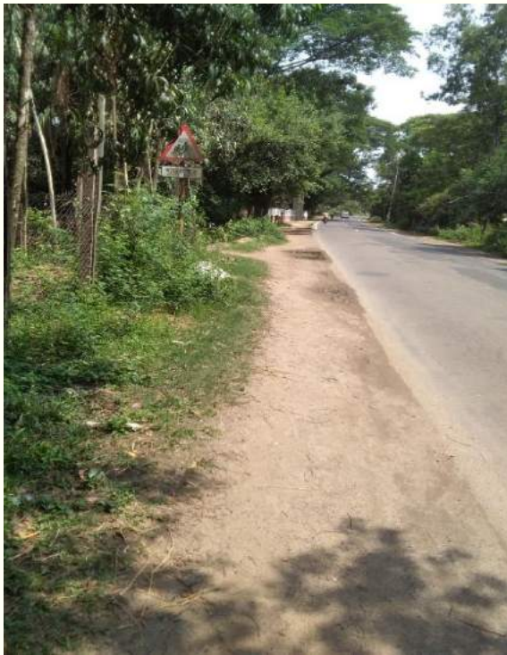
Less visible road sign at Ch.+295 to Ch.+297
