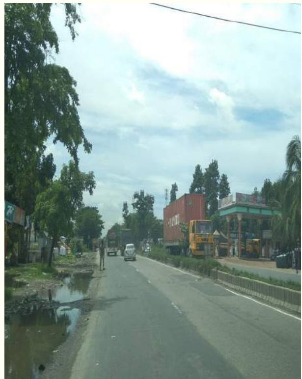
Waterlogged roadside within Ch.+25 to Ch.+27
