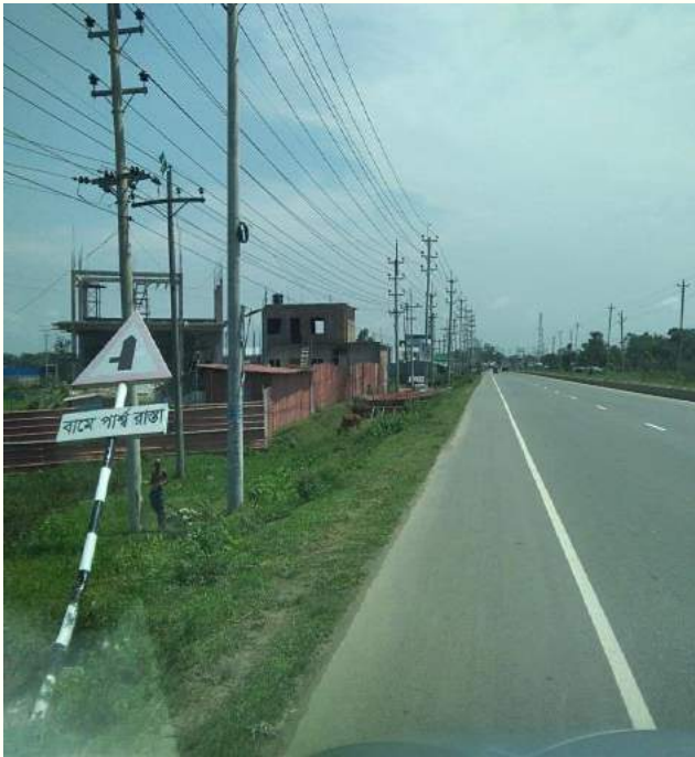
Disturbed sign post within Ch.+75.5 to Ch.+77.5
