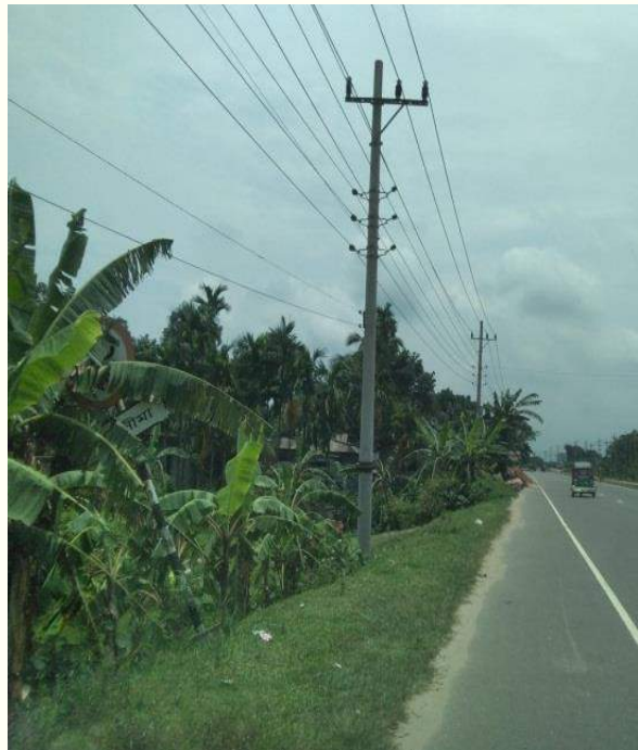
Disturbed & not visible sign post within Ch.+101.5 to Ch.+103.5
