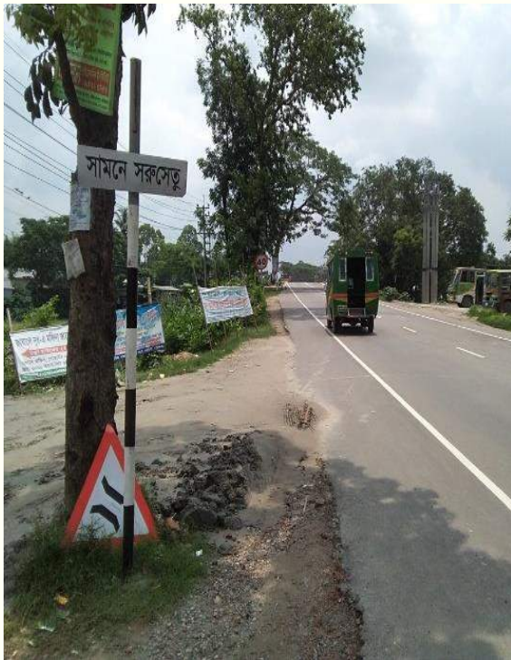
Disturbed road sign within Ch.+42 to Ch.+44
