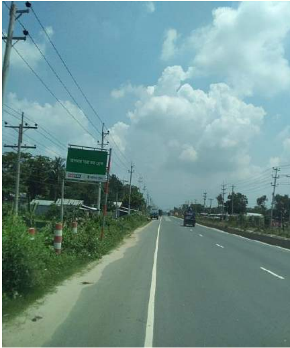
Roadside bushes within Ch.+63.6 to Ch.+65.6
