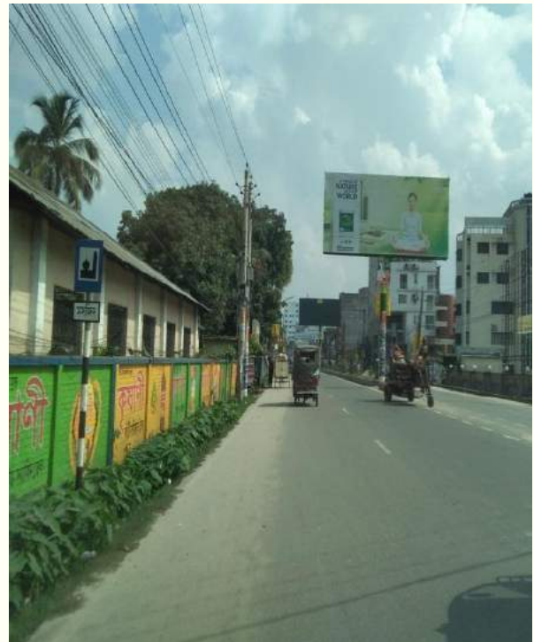
Roadside electric pole & faded road marking within Ch.+107.5 to Ch.+109.5
