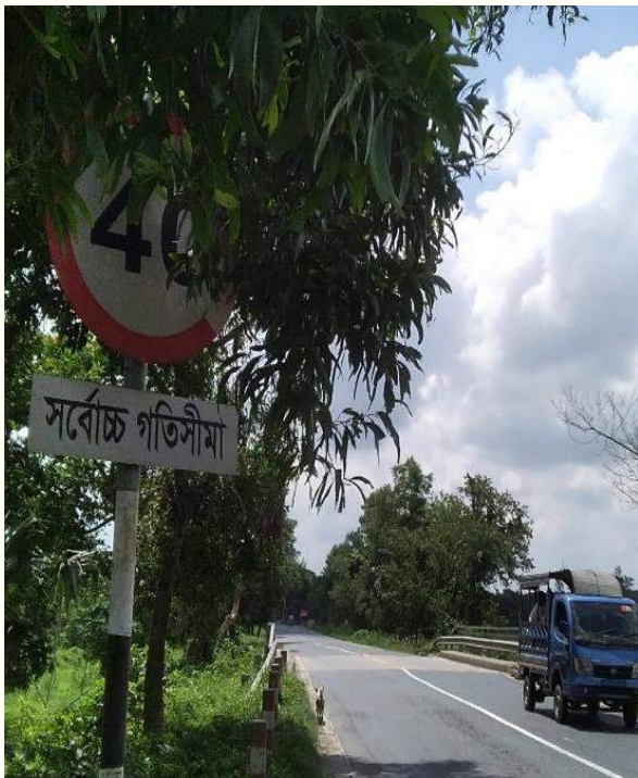
Less visible road sign within Ch.+58 to Ch.+60
