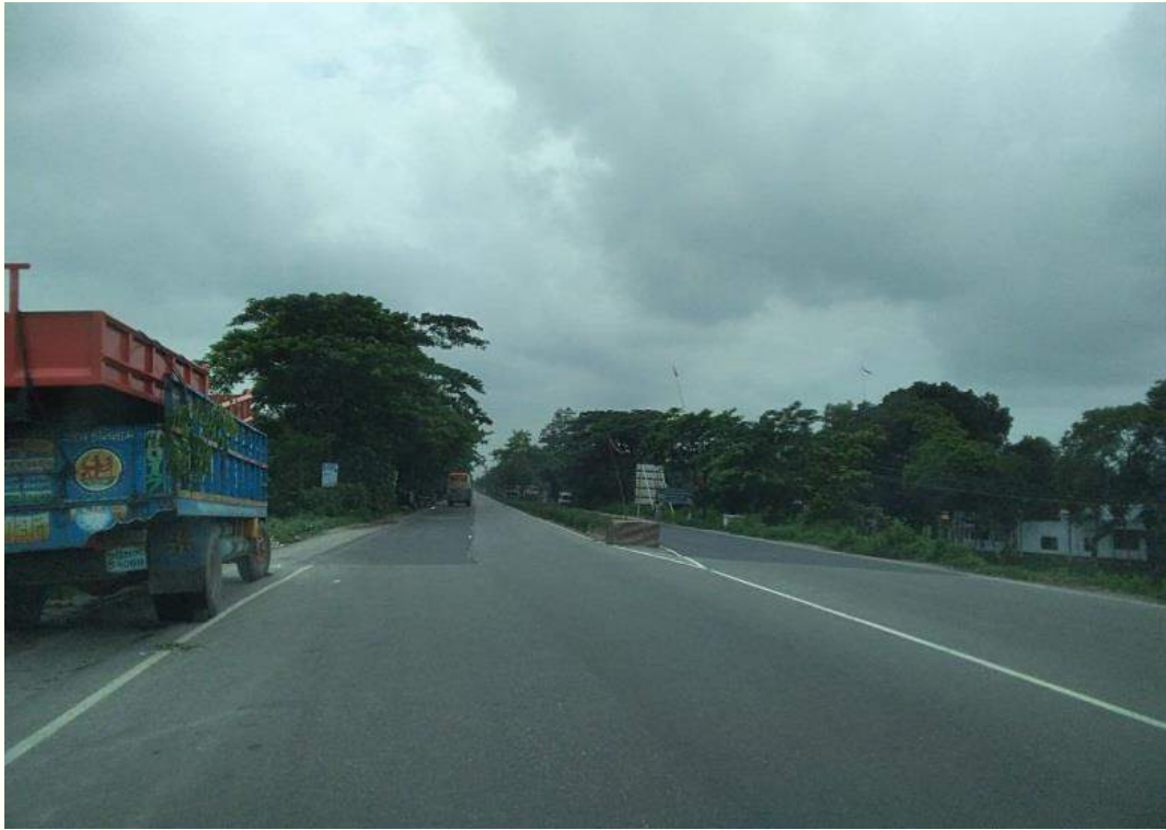
Hazardous median protection block within Ch.+35 to Ch.+37
