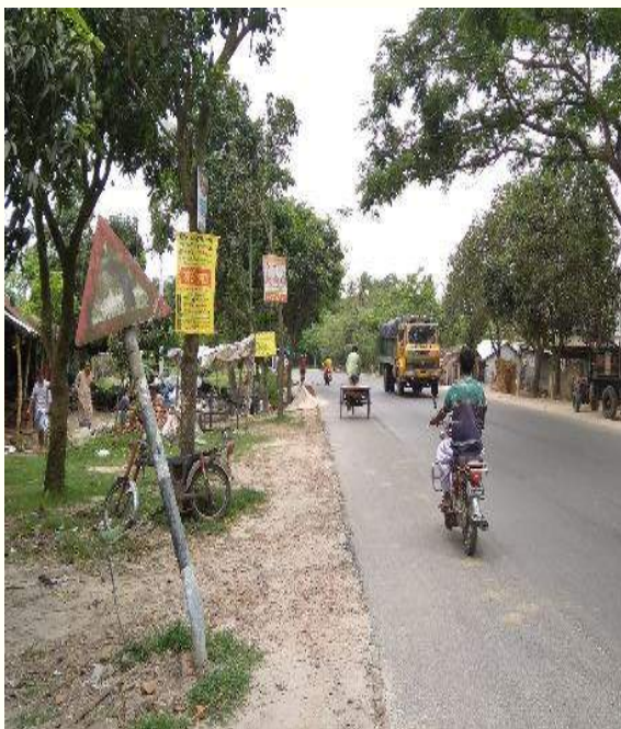
Disturbed road sign within Ch.+110 to Ch.+112
