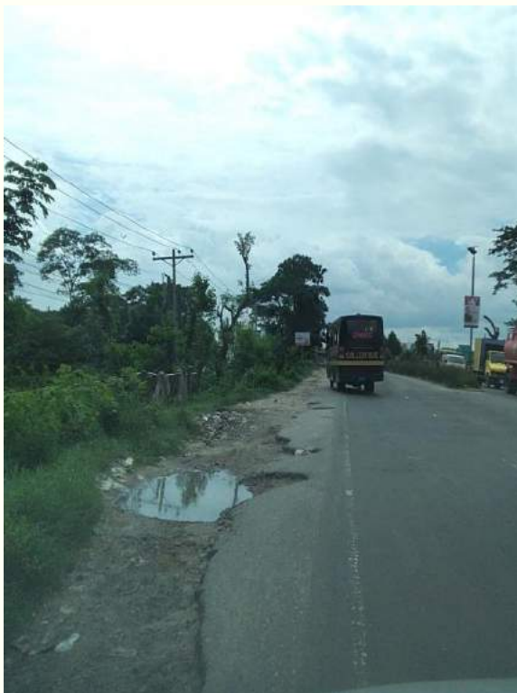
Broken shoulder and waterlogging within Ch.+19 to Ch.+21
