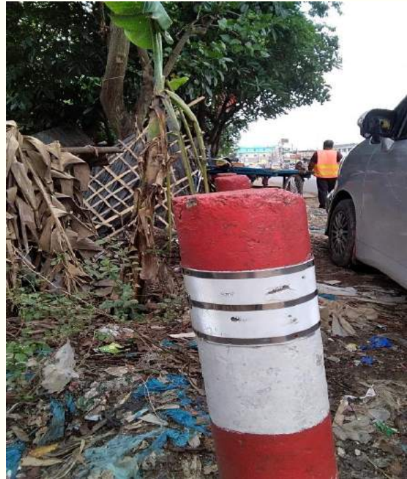
Disturbed concrete pole at Ch.+ 355 to Ch.+357
