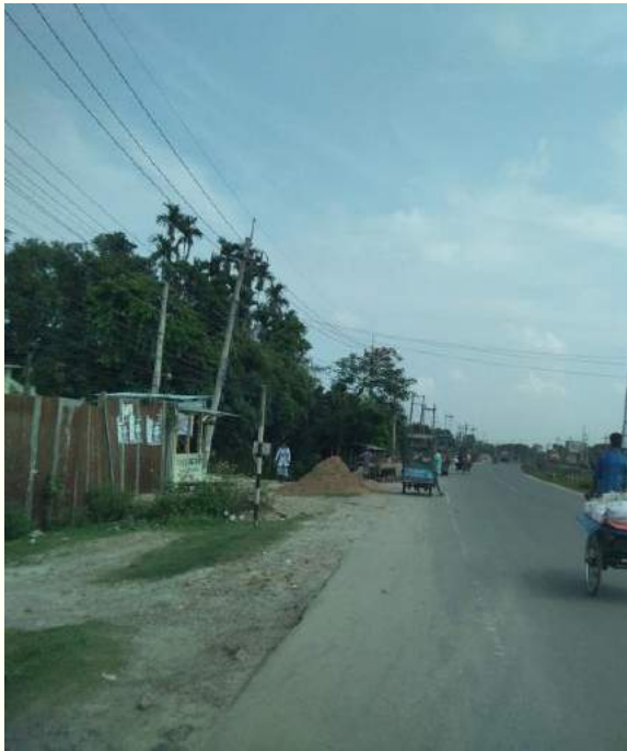
Faded road marking within Ch.+87.5 to Ch.+89.5
