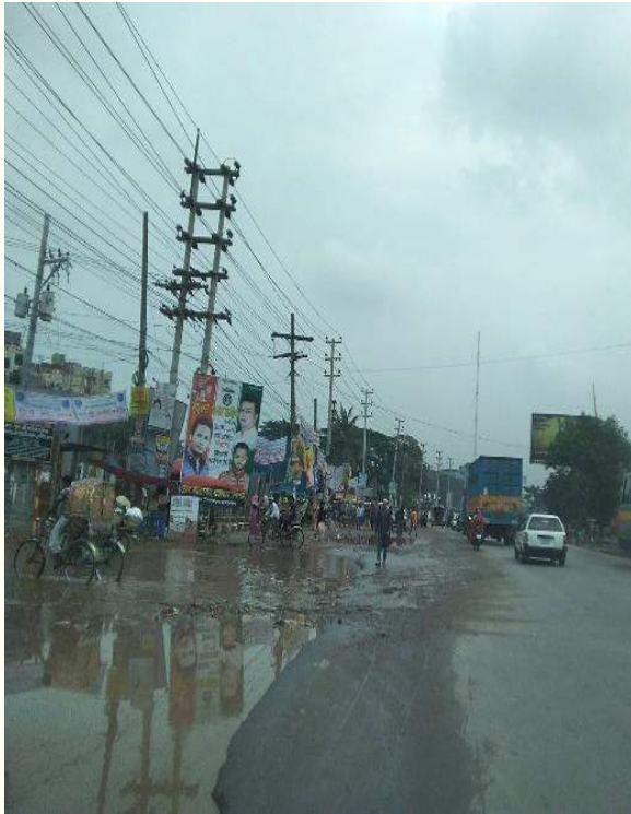
Water logging within Ch.+14 to Ch.+16
