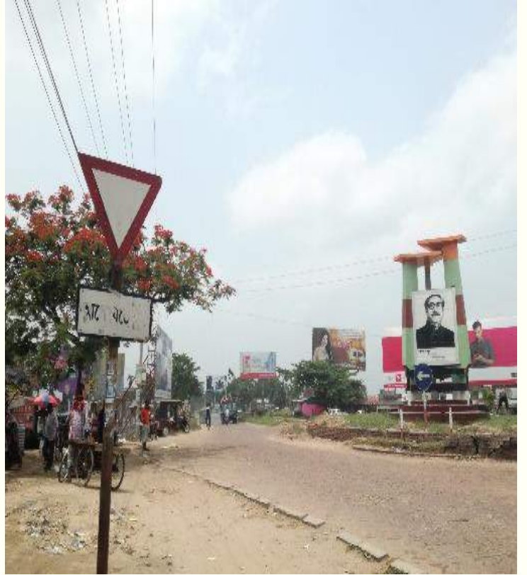
Faded sign within Ch.+84 to Ch.+86
