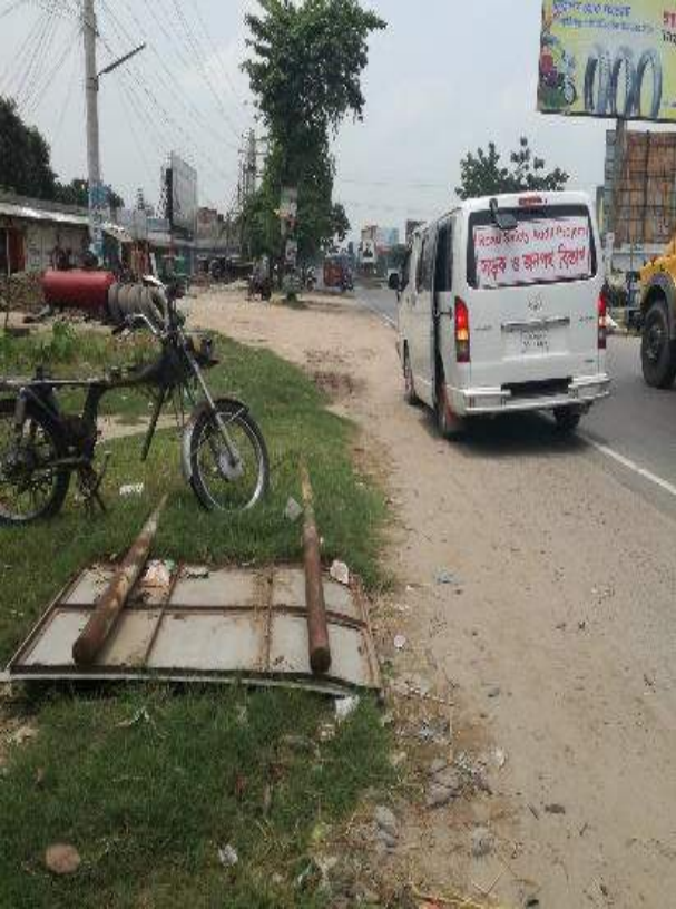
Broken sign within Ch.+84 to Ch.+86
