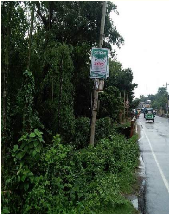
Roadside bushes occupying earthen shoulder at Ch.+ 272 to Ch.+274
