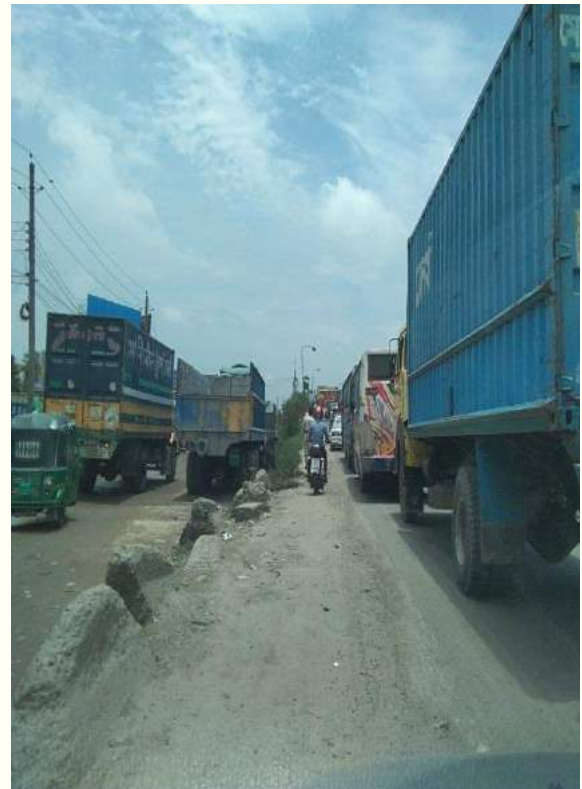
Risky and broken blocks on middle road Ch.+ 9 to Ch.+11
