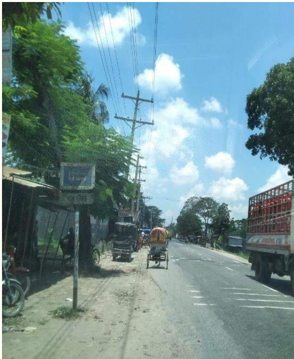
Less visible road sign within Ch.+64 to Ch.+66
