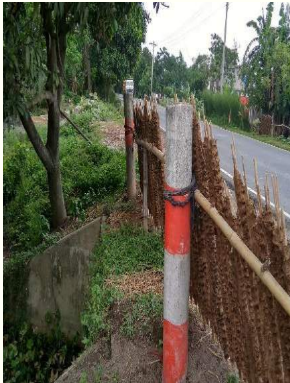
Unauthorized road side activities within Ch.+72 to Ch.+74
