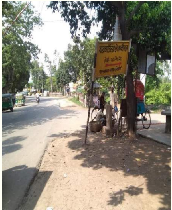
Unknown road sign within clear zone at Ch.+ 297 to Ch.+299
