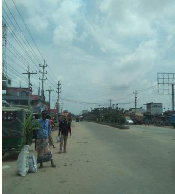
No road marking & unauthorized parking within Ch.+99.5to Ch.+101.5
