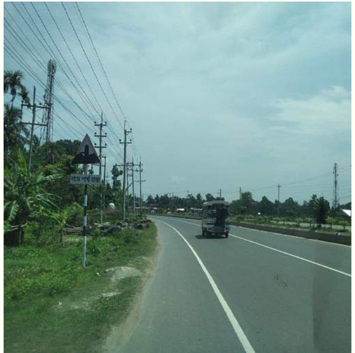
Disturbed sign post within Ch.+77.5 to Ch.+79.5
