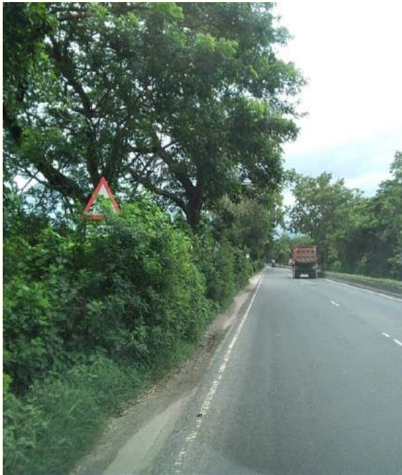
Invisible road sign within Ch.+29 to Ch.+31
