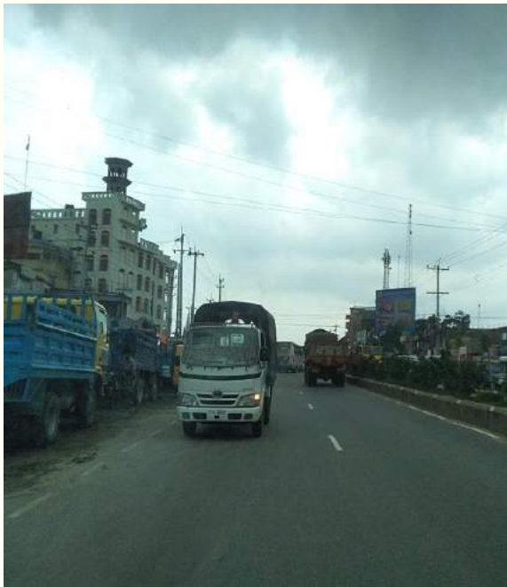
Contra flow within Ch.+59.6 to Ch.+61.6
