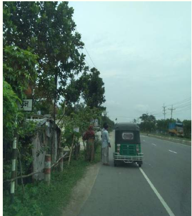
Invisible sign post & insufficient earthen shoulder within Ch.+93.5 to Ch.+95.5
