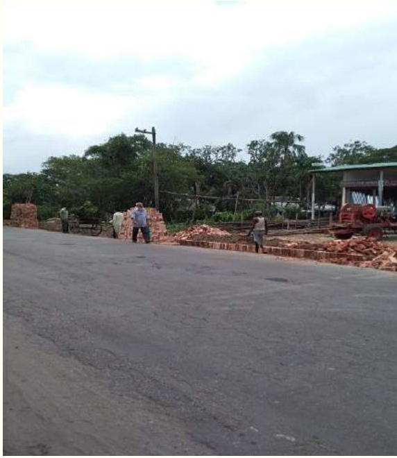
Illegal roadside activity within Ch.+ 252.5 to Ch.+255
