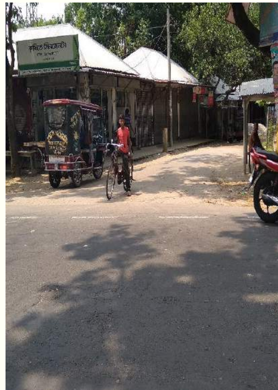
Side road without proper treatment within Ch.+ 30 to Ch.+32
