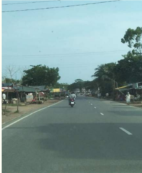
Unauthorized roadside business within clear zone at Ch.+ 271 to Ch.+272
