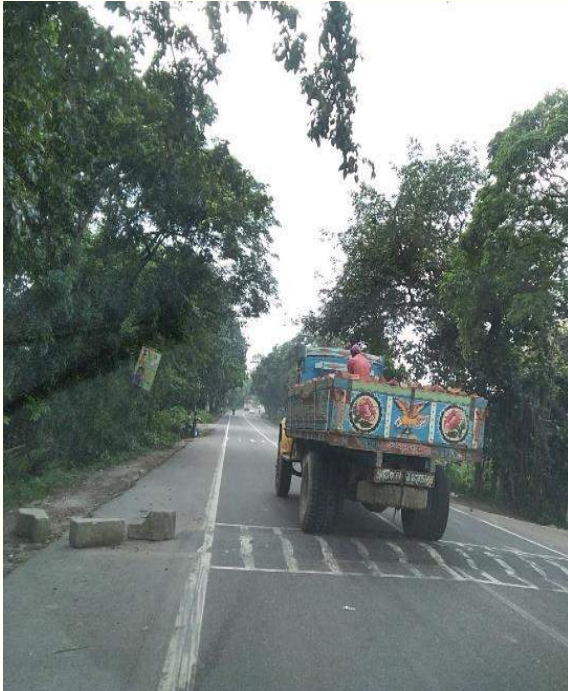
Risky concrete block placed within Ch.+42 to Ch.+44
