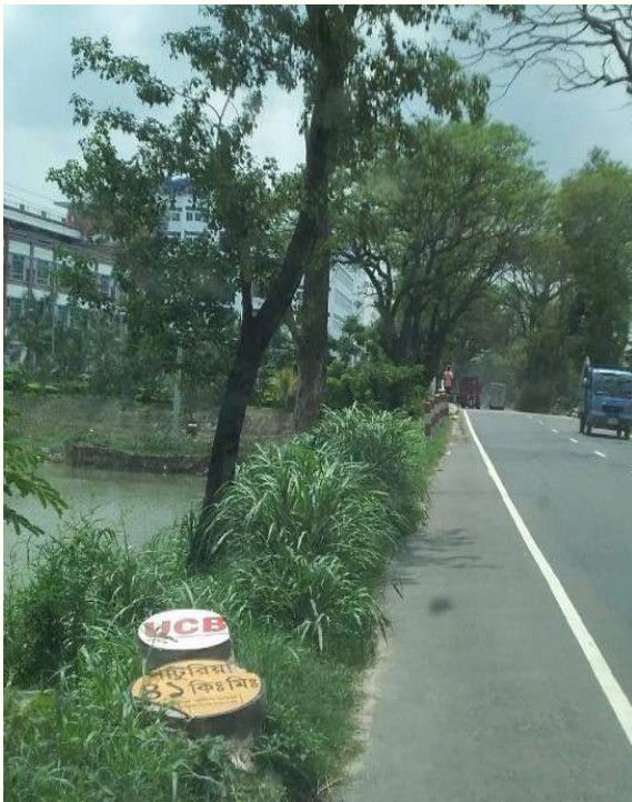
Disturbed, unknown km post within Ch.+36 to Ch.+38
