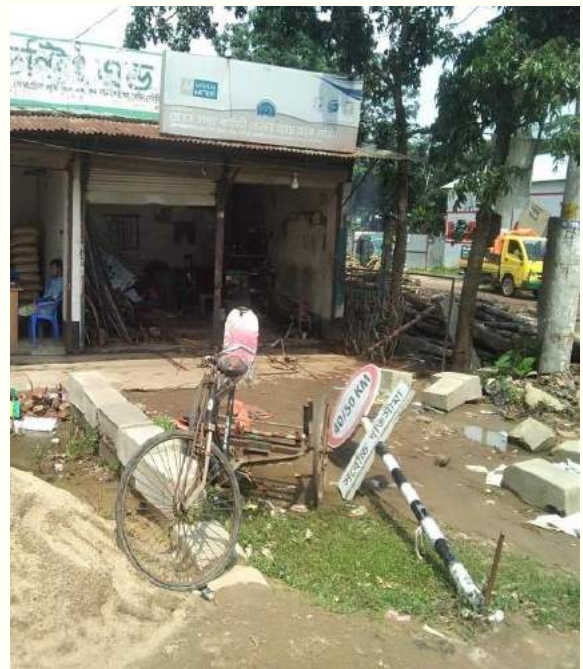
Disturbed & broken sign within Ch.+53.6 to Ch.+55.6
