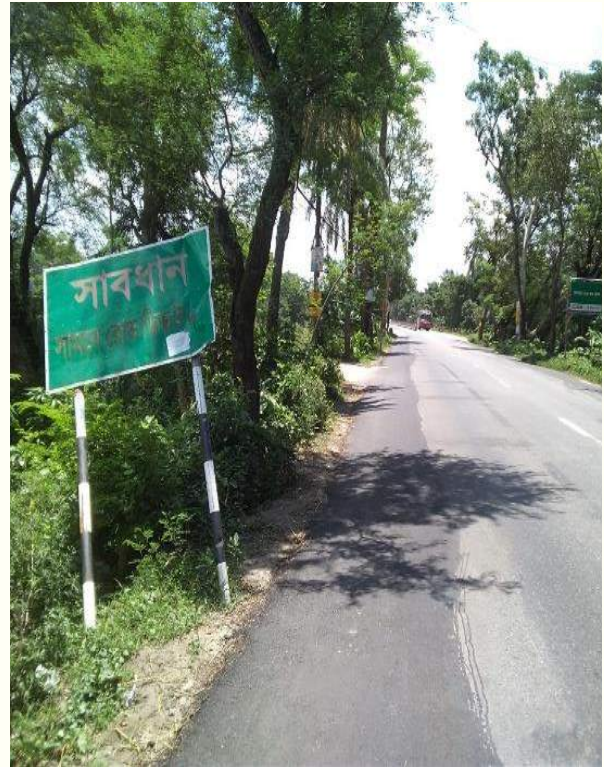
Disturbed road sign within Ch.+62 to Ch.+64
