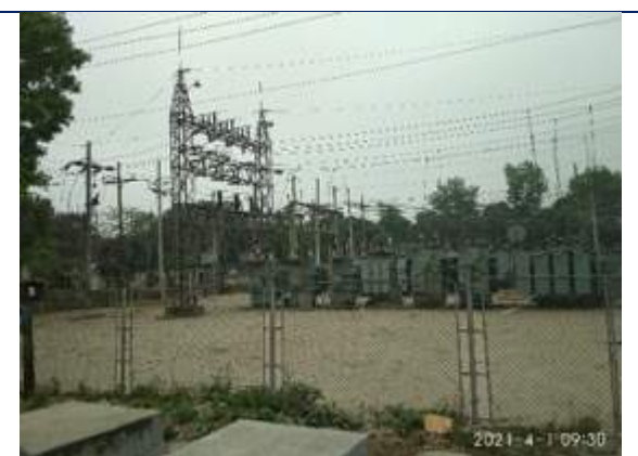
substation site at uttar Gobindopur, Dinajpur PBS
