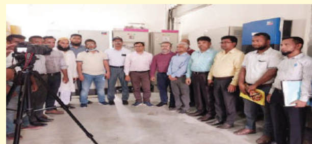
Figure: 2 : BREB's Net Metering Station
