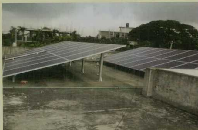
Figure 2: 10 kWp rooftop solar plant with Net metering at Narayanganj PBS-2
