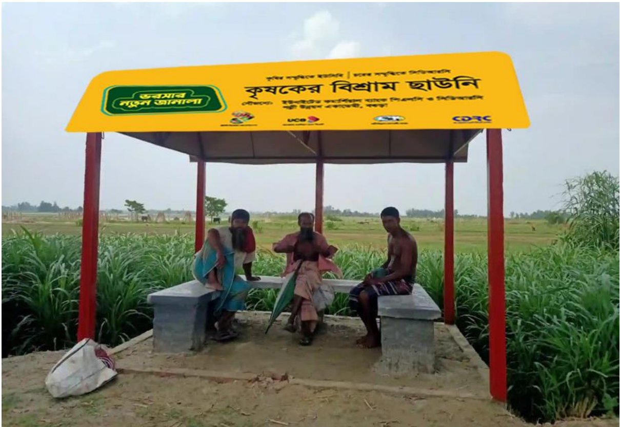
3. A Farers Resting place was constructed in Nayapara Char, Sariakandi, Bogura.
