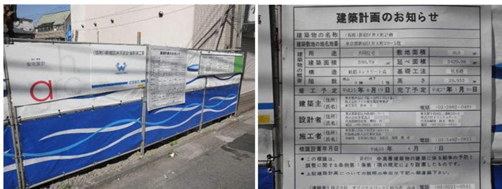
Figure 4 Outline and important information on construction work must be shown at the construction site in Japan such as use/occupancy of buildings, number of stories, height, floor area, coverage area of buildings, name of the owners, name of designers, name of contractors, etc.. If neighboring people are skeptical, he/she can inform the regulatory authority.
