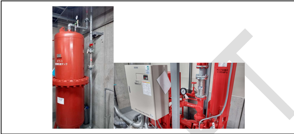
Figure III-8: Example of Foam extinguishing system
