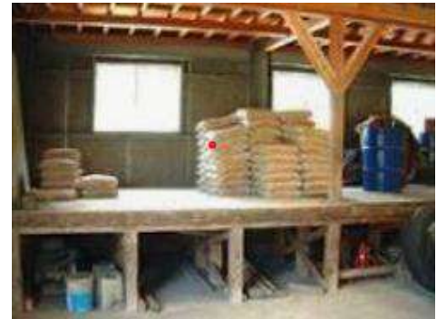
Figure 2-22 storing of cement
