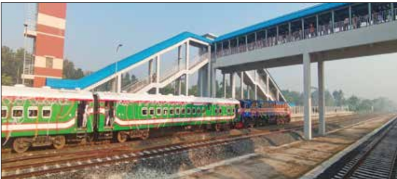
Kashiani Junction Station built under the Padma Bridge Rail Link Project.
