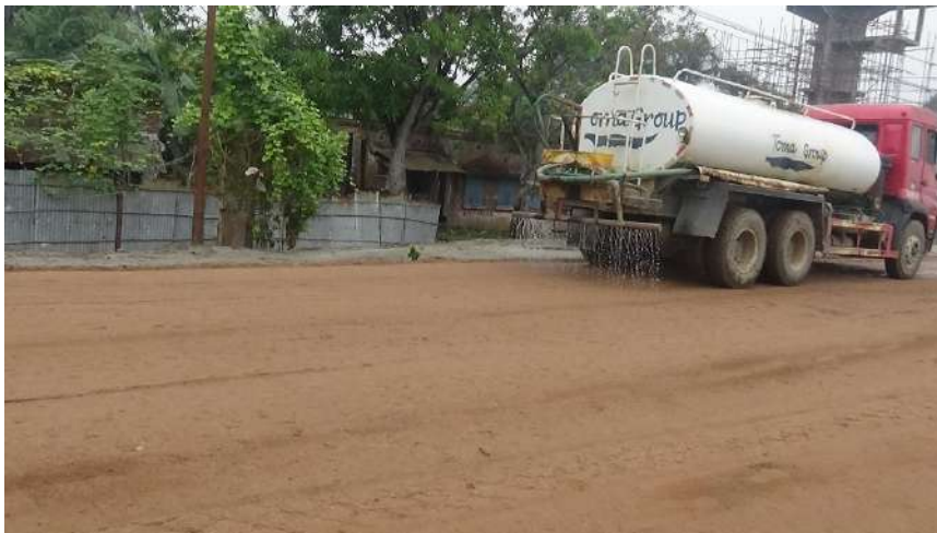
Plate 5. Photograph of watering of unpaved track embankments at Akhaura yard. Picture taken on 15 November 2021.
