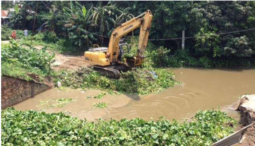
Plate 7. Photograph of clearing waterway of Bridge No. 1 at the Akhaura Station Yard. Picture taken on 8 July 2021.
