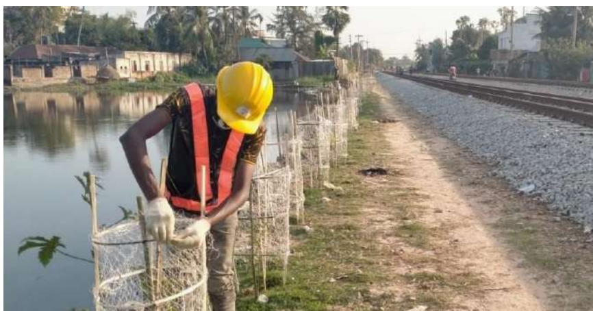
Plate 25. Individual fencing installed at planted saplings at chainage km151+000. Photograph taken on 06 December 2021.
