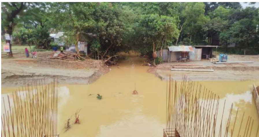
Plate 9. Photograph of clearing waterway as part of the construction of culvert No. 256. Picture taken on 8 December 2021.
