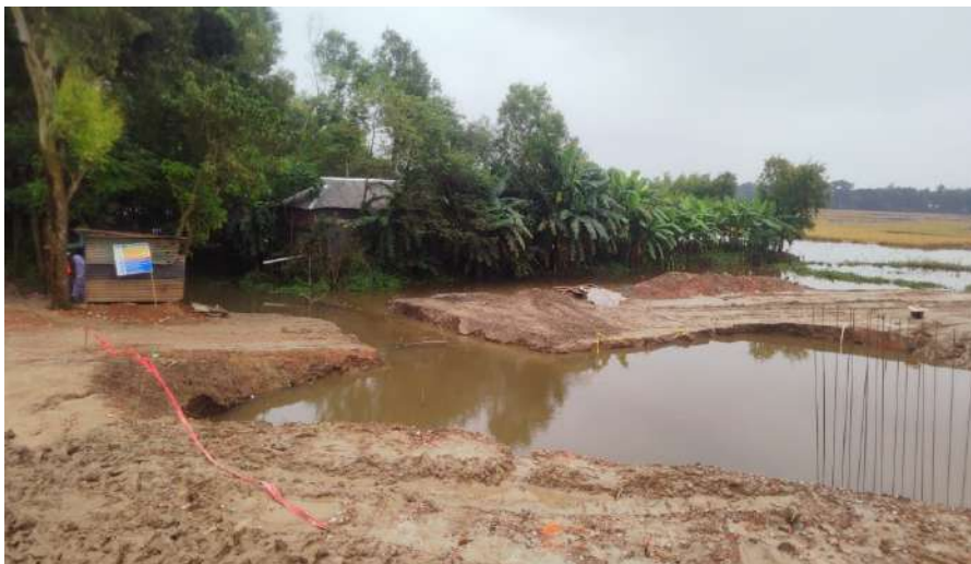
Plate 8. Photograph of clearing waterway as part of the construction of culvert No. 258. Picture taken on 22 December 2021.
