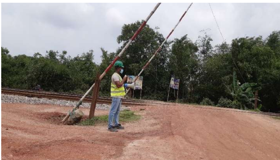
Plate 18. Gateman deployed at a temporary rail level crossing where active construction work is on-going, to regulate the movement of traffic Picture taken on 6 August 2021.
