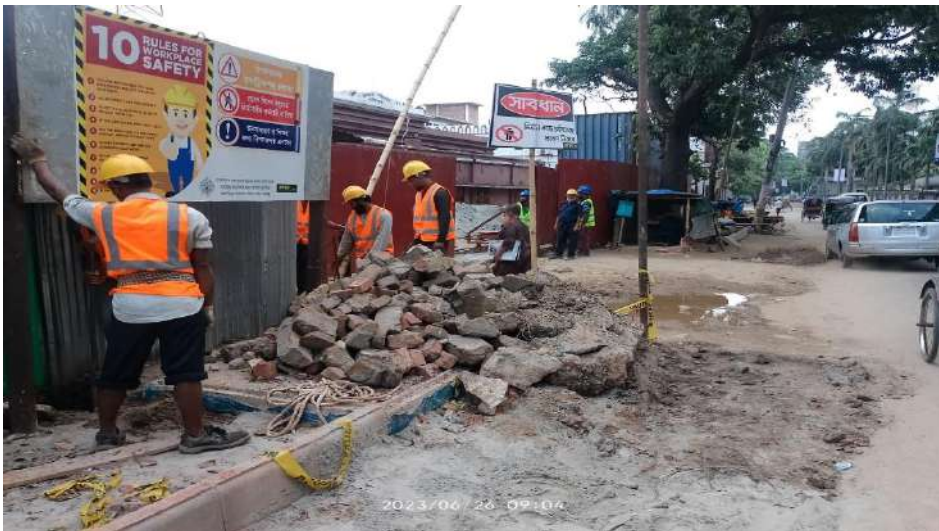
Plate 32. Safety informative signs installed at the front perimeter wall of EMO Building construction site. Debris also temporarily piled for collection by licensed contractor. Photograph taken on 26 July 2023.
