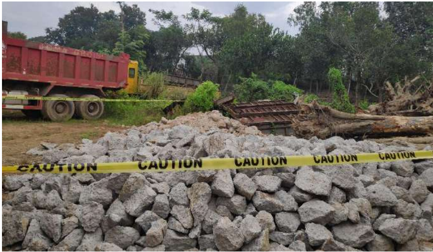
Plate 7. Photograph of excess construction materials, excavation spoils and cut trees deposited in temporary storage area prior to disposal in LGU authorized sites, on 16 November 2023
