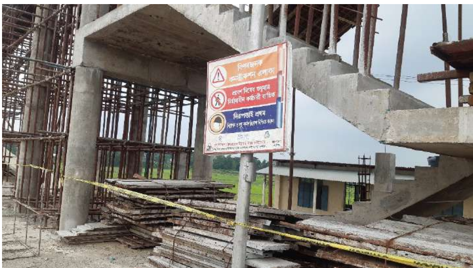
Plate 18. Informative signs and yellow table placed at construction site to warn workers, commuters and pedestrians of possible dangers that may occur at the Gangasagar train station construction site. Picture taken on 9 June 2022.
