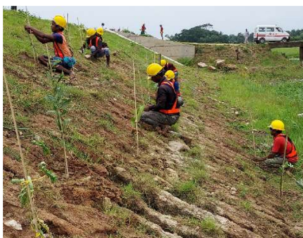
Plate 4. Tree plantation workers install bamboo sticks as support to the newly planted tree saplings at Section 3 track embankment slopes.
