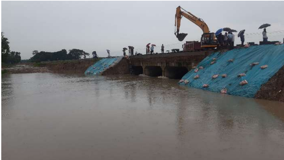
Plate 7. Photograph of clearing waterway. Temporary cover for newly established embankment to avoid soil erosion. Sodding will be done later. Picture taken on 18 June 2022.
