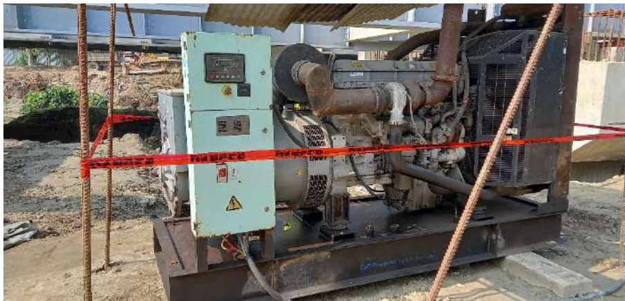
Plate 14. Photograph of the Quasba Office electric power generator with fuel tank and tin roofing. Picture taken on 9 February 2022.
