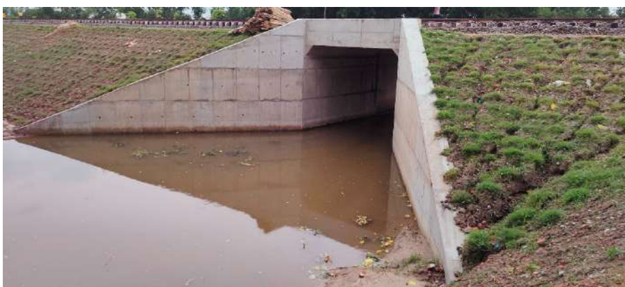
Plate 9. Photograph of newly constructed box culvert with sodded approach to help prevent soil erosion that may block the waterway. Picture taken on 25 June 2022.
