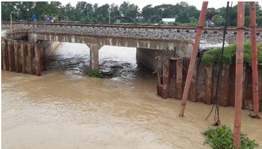
Plate 8. Newly constructed 2 cell box culvert cleared of debris to allow free flow of flood waters. Picture taken on 19 June 2022..
